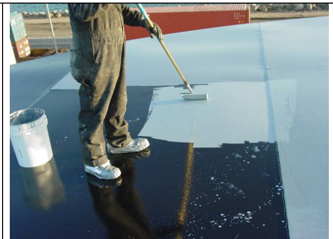
FIGURE 14. AZT Topcoat Applied by Rollers on Tank 2001 roof.
