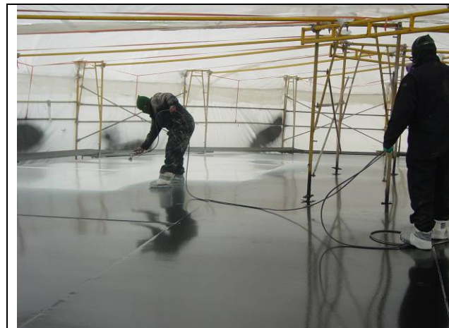
FIGURE 13. Spray application of LVBC Barrier Coating on Tank 2003 roof.
