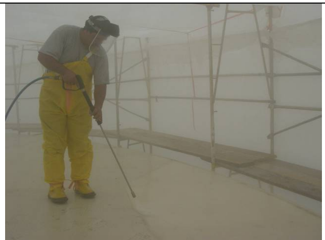
FIGURE 12. Surface Preparation by Water Blasting.
