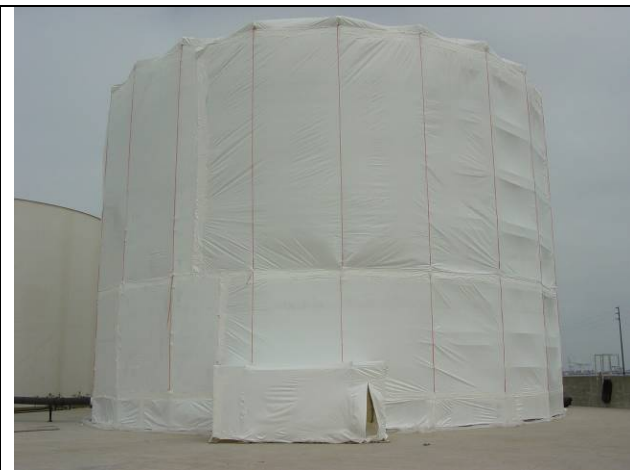
FIGURE 11. Containment Plastic over Scaffolding on Tank 2003.
