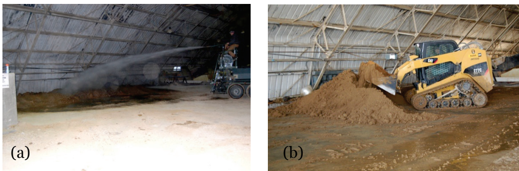
Figure 9. Soil preparation: a) wetting soil using a hydro-seeder and b) mixing soil using a skid steer.
