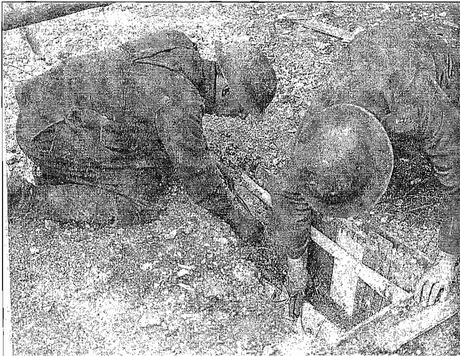
Figure 15. Royal Engineers Working on an Improvised Electrically Initiated Mine
