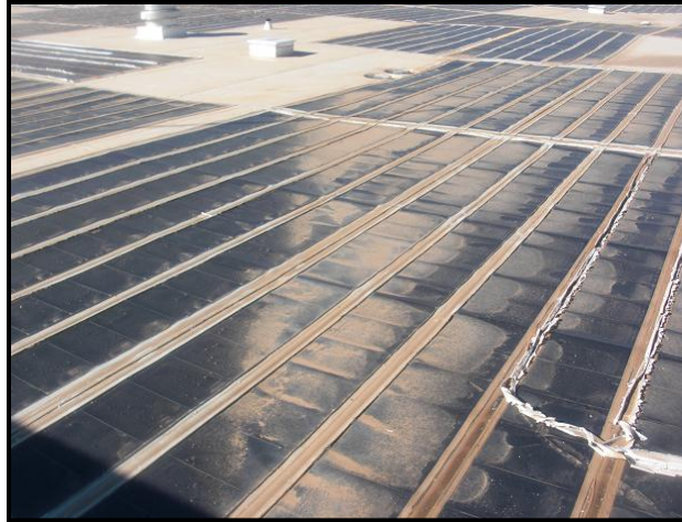
Figure-22: Tape deterioration and soiling of the PV system at Site I (Luke AFB).
