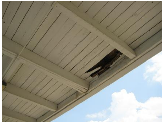
Figure 3 Building 515 Rotten Section
