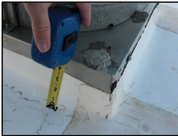
Figure-43: Photo of Site III (MCAS Yuma) exhaust vent with insufficient flashing height.
