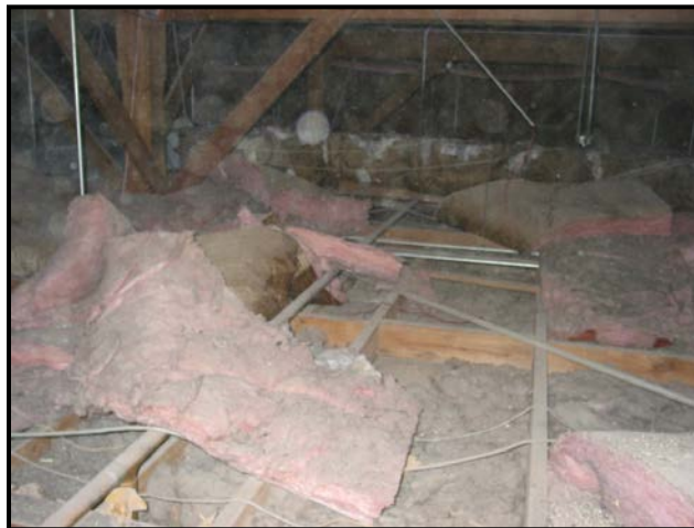
Figure-12: Attic space of Building 228 at Site III (MCAS Yuma) showing poor insulation.
