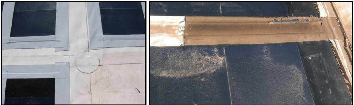
Figure-21: Tape solution soon after it was applied (left) and deterioration later that year (right) Site I (Luke AFB).
