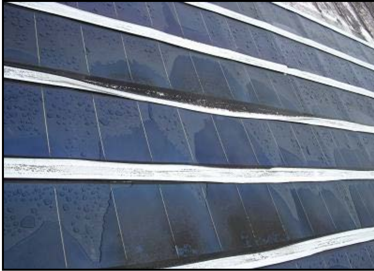
Figure-45: Water ponding due to the failing tape and PV module orientation. Mold growth in the upper right corner.
