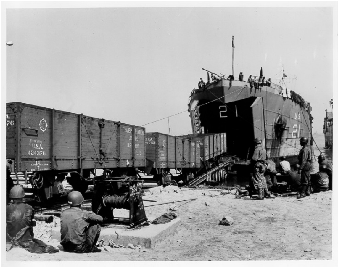
Figure 16. LST-21 Off-loading Railroad Cars
