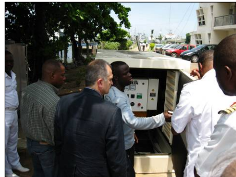
Nigeria - Support Generator
