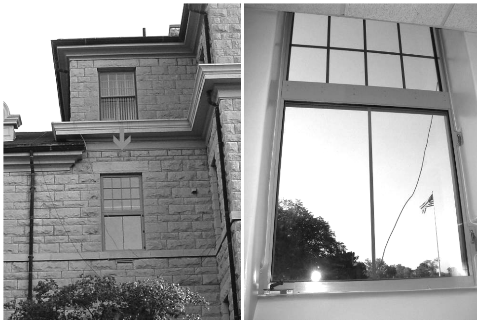
Figure 41. Casement window manufactured to resemble a double-hung unit (left). Challenges of incorporating new casement hardware into fenestration designed for double-hung units (right). The interior wall was carved out to provide clearance for the casement cranks and locks (DA 2005).
