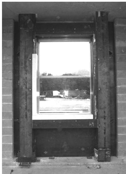
Figure 44. Window-flanking bracing transfers loads to floors and ceilings (PDC 2004).
