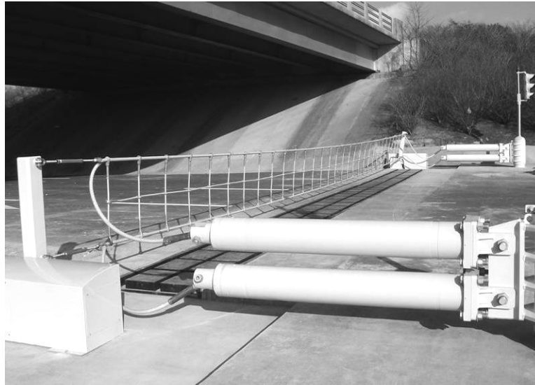
Figure 10. Above-grade components of vehicle net barriers may create a visual challenge when installed a historic landscape (Universal 2005).
