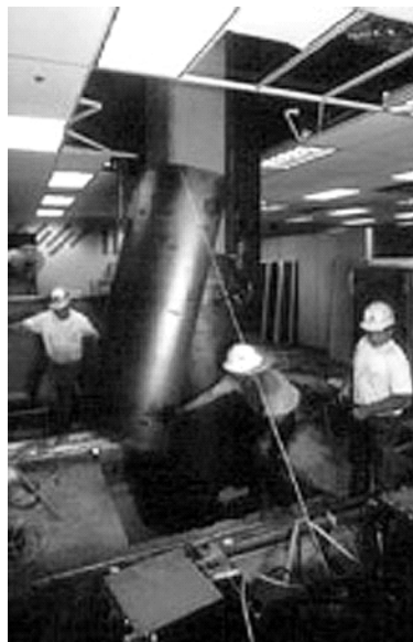
Figure 17. Seismic application of a steel jacket on an existing concrete column (Morley Builders 1997).
