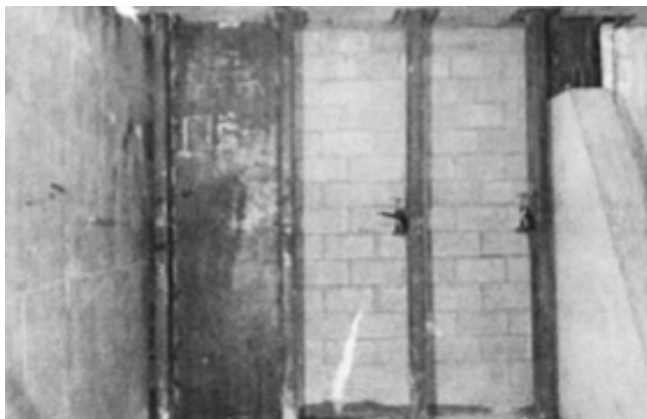
Figure 24. Steel column and plate application (Ward 2004).
