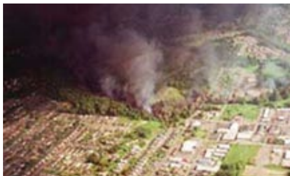
Figure 9 - Gas Pipeline Explosion Caused by SCADA Malfunction
