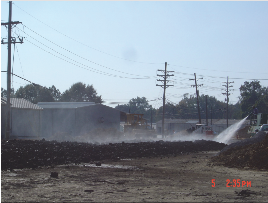
Figure 19. Adding water to the subgrade material.
