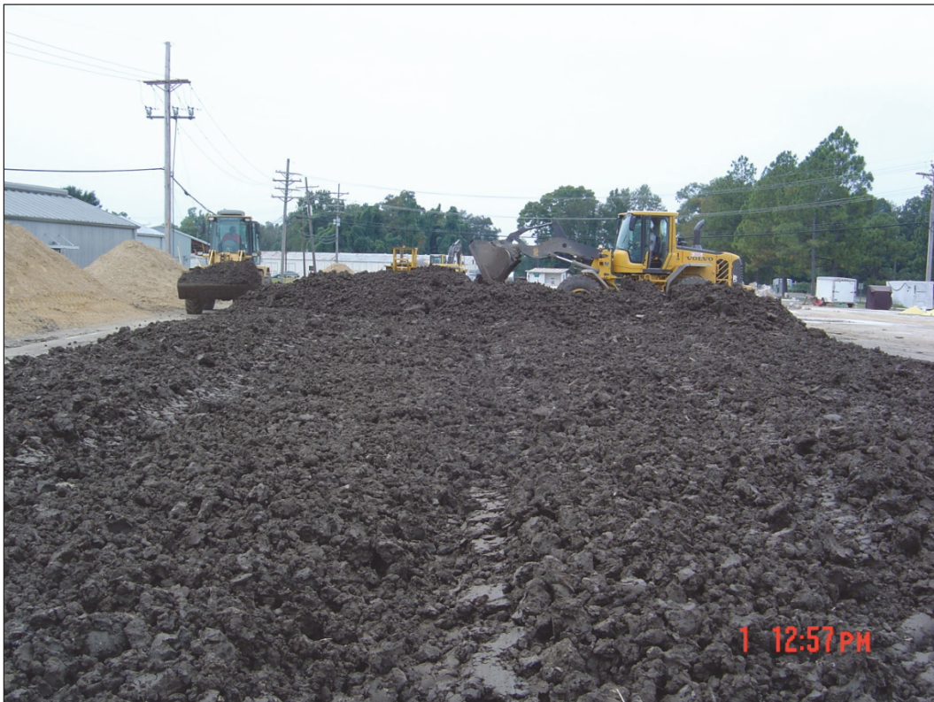
Figure 20. Subgrade material processing.
