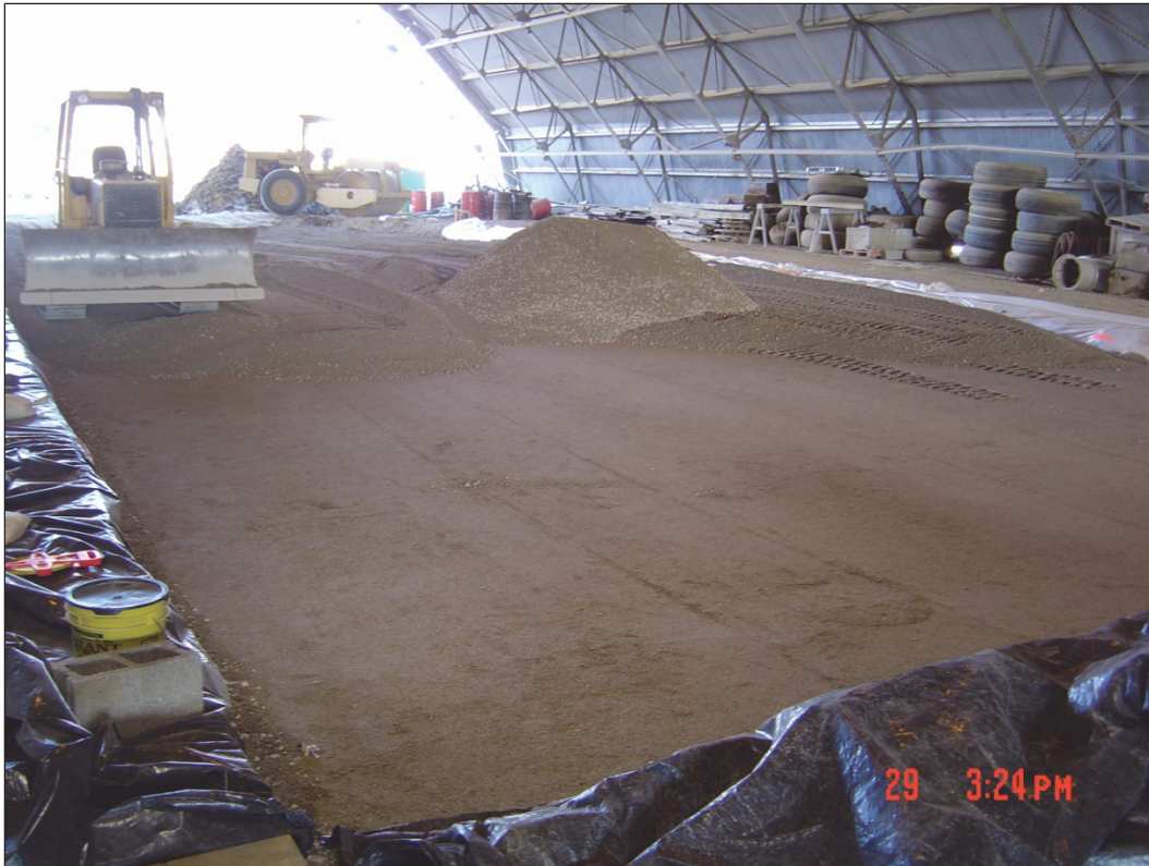
Figure 25. Subbase placement activities.
