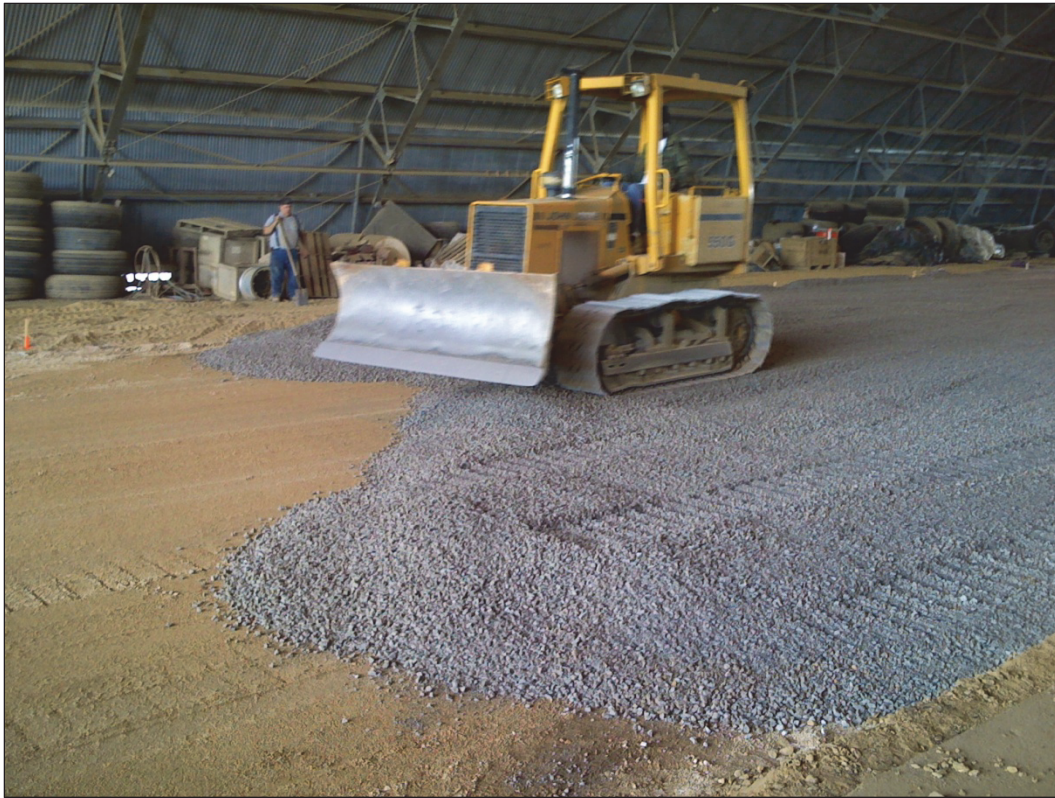
Figure 27. Base layer placement.
