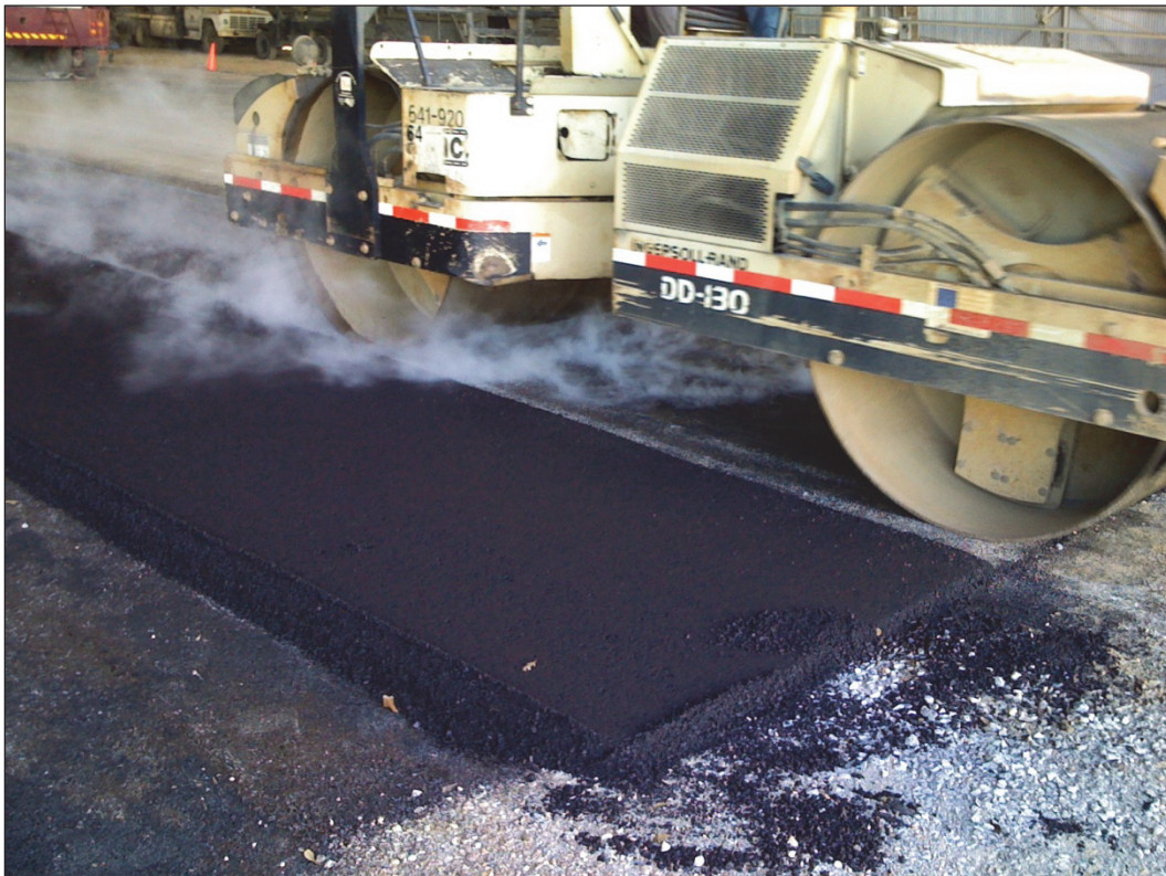
Figure 30. Paving operations, break-down rolling.
