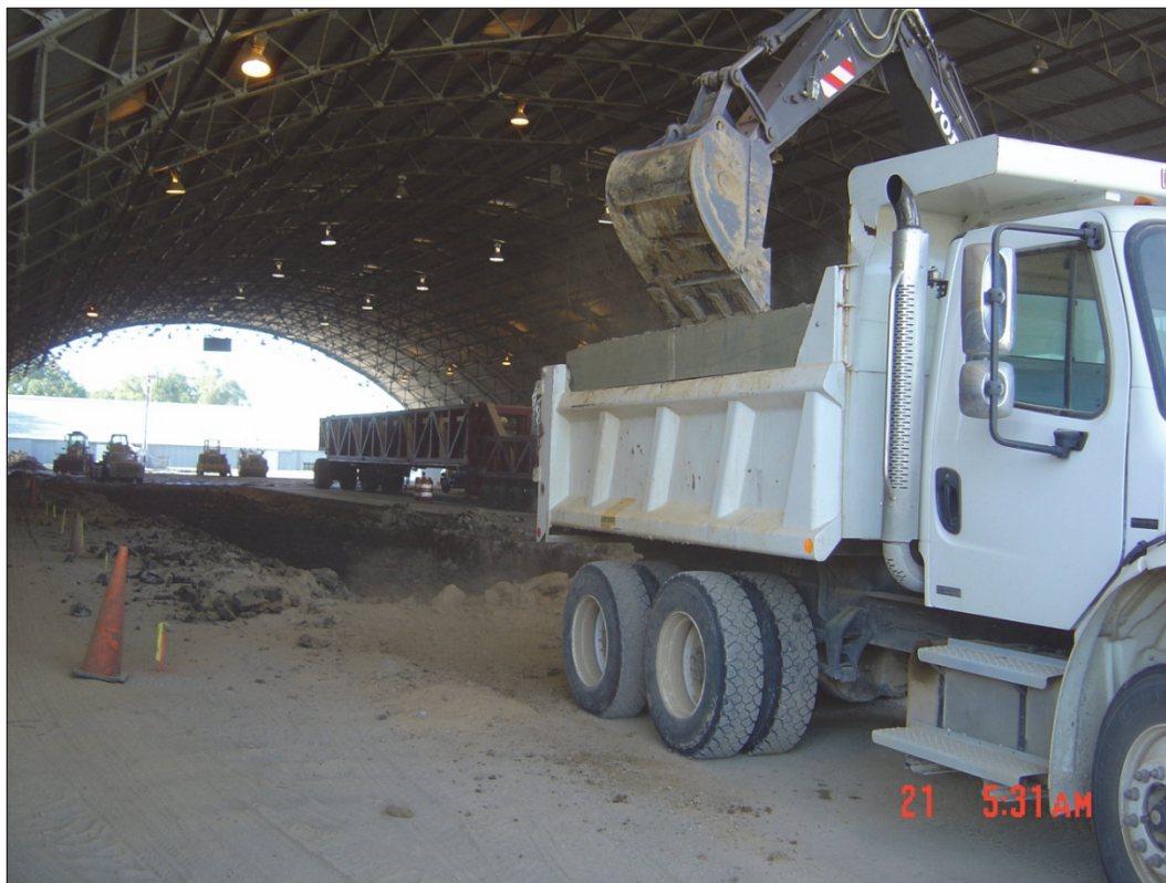
Figure 18. Test section excavation.
