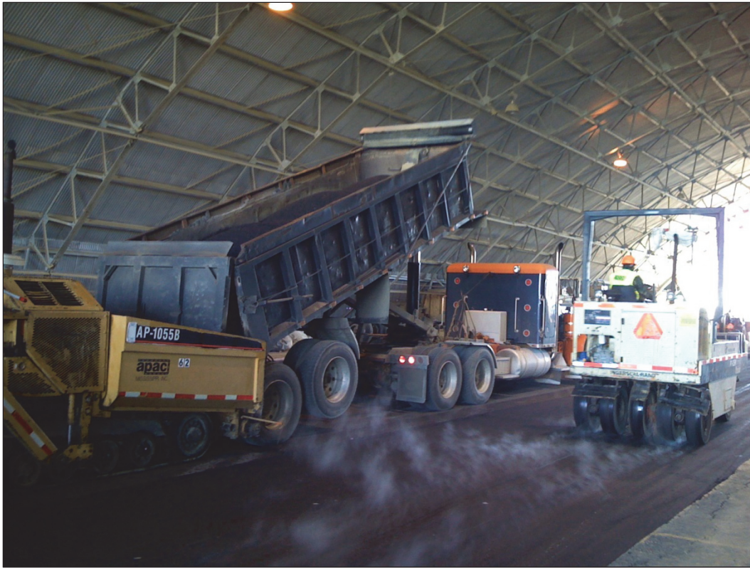
Figure 31. Paving operations, rubber-tire roller compaction.
