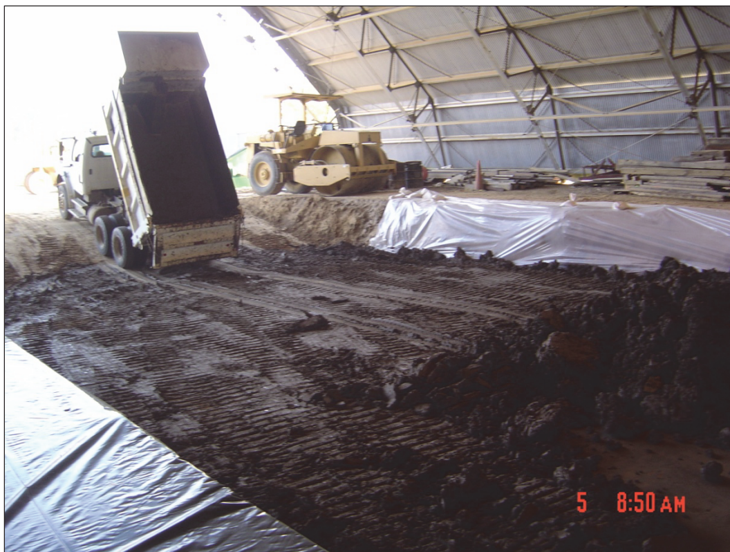
Figure 21. Subgrade material placement.
