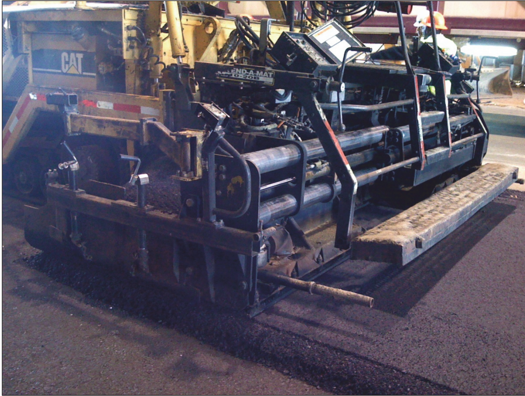
Figure 29. Paving operations, mat placement.
