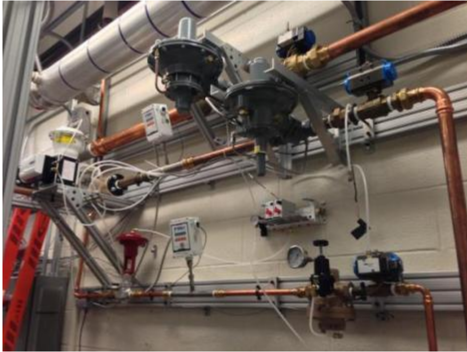
Figure D.7: 0.75", 1.5", and 3" air lines
