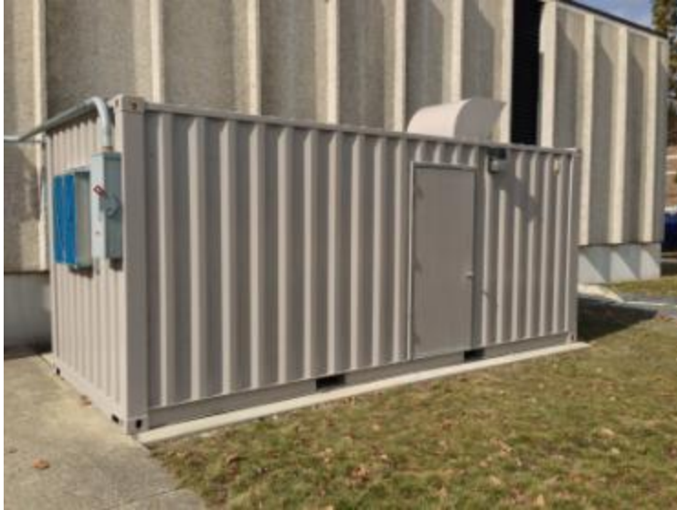
Figure D.1: Air compressor housing outside COAL lab
