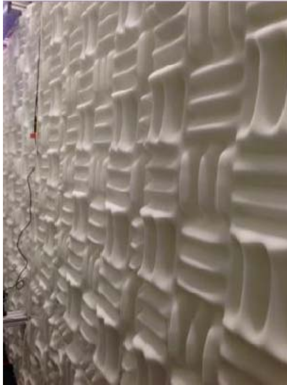
Figure B.1: Sound absorbing panels
