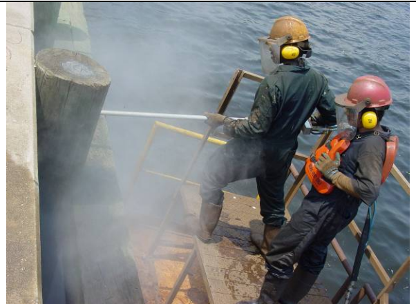
FIGURE 16. Pensacola steel sheet pile surface preparation.
