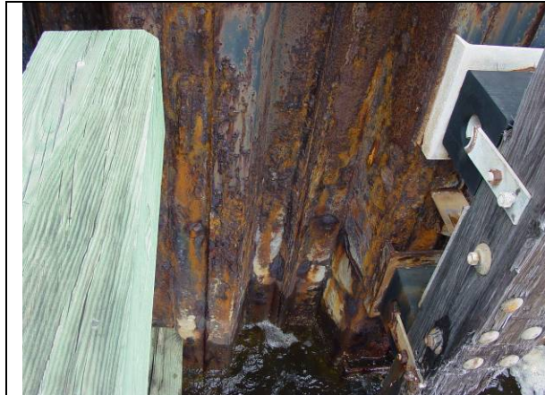
FIGURE 15. Typical corrosion on Pensacola steel sheet pile before surface preparation.
