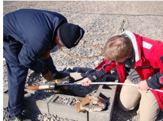
Figure 20. Val and Garry feed the PEX tubing into the pipe to melt the ice securing the cables.
