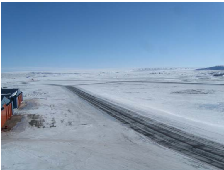
Figure 15. View from the tower April 2011, looking east to the 26 end of the runway. The faded and dark nature of the paint is very evident against the backdrop of white snow.
