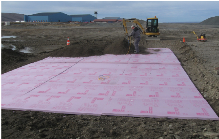
Figure 25. XPS insulation placed at base level for the test embankment.
