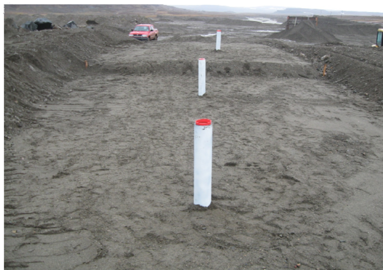
Figure 26. Completed test embankment with thermal buffer fill piled around the test.
