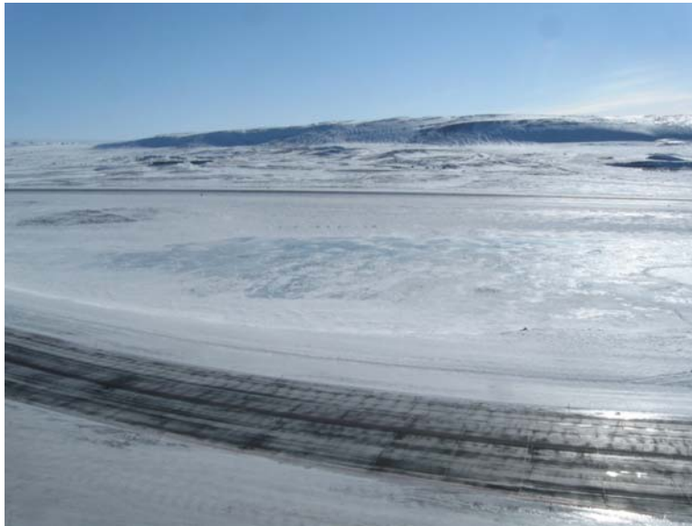
Figure 16. View from the tower in April 2011, looking directly south over Lake Eddy. The dark colored runway and taxiway are visible.
