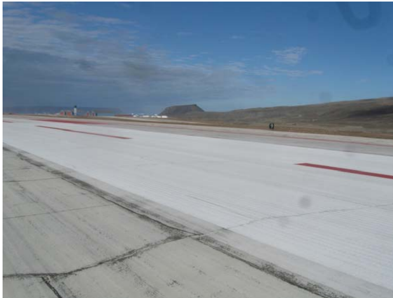
Figure 20. Bright white runway at 91+00. Albedo measured at 0.58 and the thaw depth measured at 3.9 ft.
