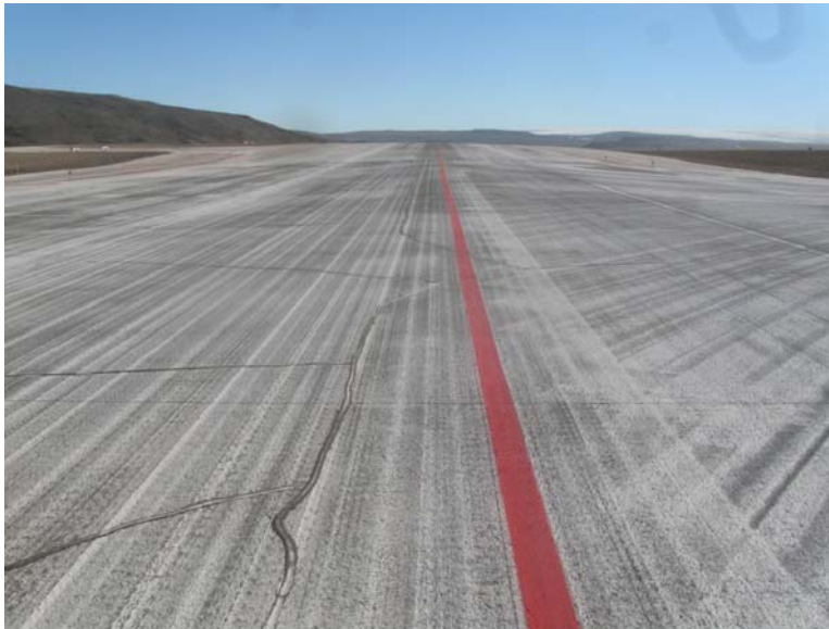
Figure 22. View east along Txwy A at Txwy Charlie. Albedo measured at 0.32. The measured thaw depth is 5.3 ft.
