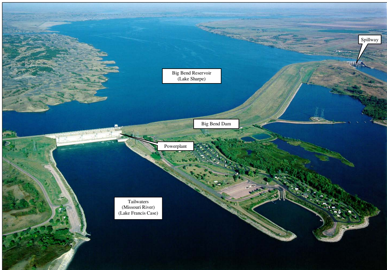
Aerial Photo of Big Bend Dam, Tailwaters and Reservoir
