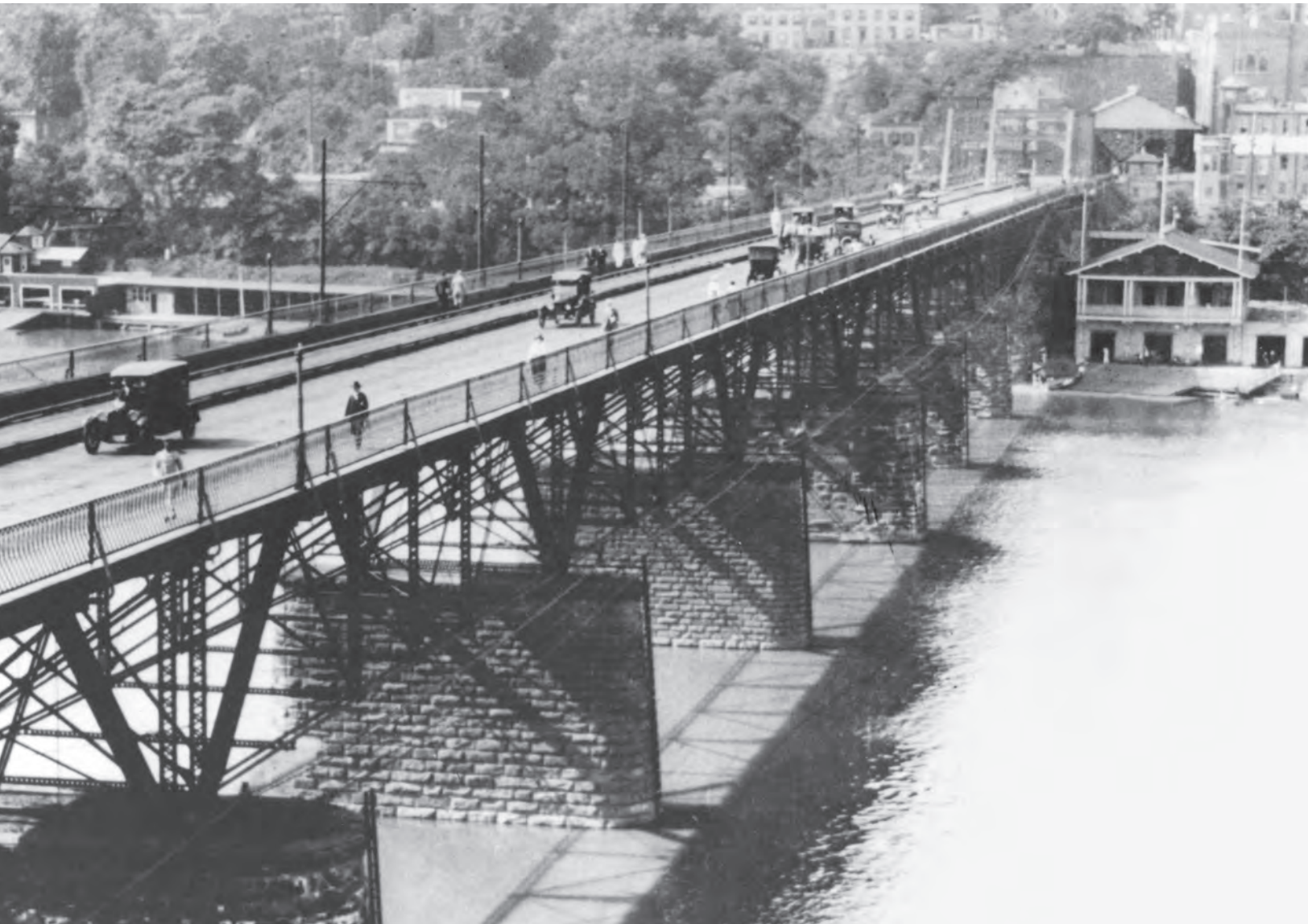
Superstructure built in 1887, supervised by Hains, on the piers of the Aqueduct Bridge between Georgetown and Rosslyn Office of History, Corps of Engineers
