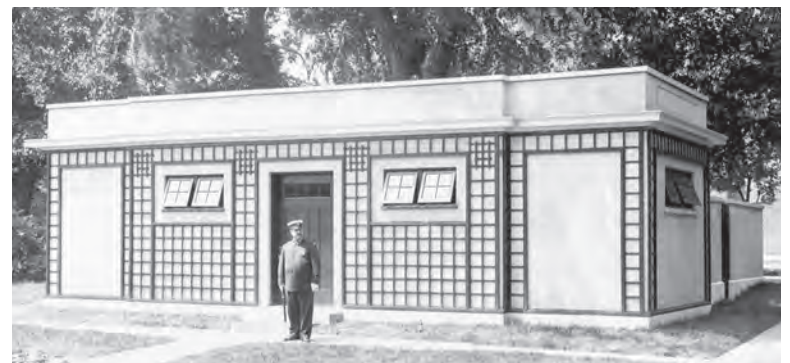
Residents facing Lafayette Square demanded a public hearing to review the placement and design of the new "gardener's lodge" in 1914. Vine-covered trellises were to obscure the building's main purpose—public restrooms. National Archives no. 42-SPB-9
