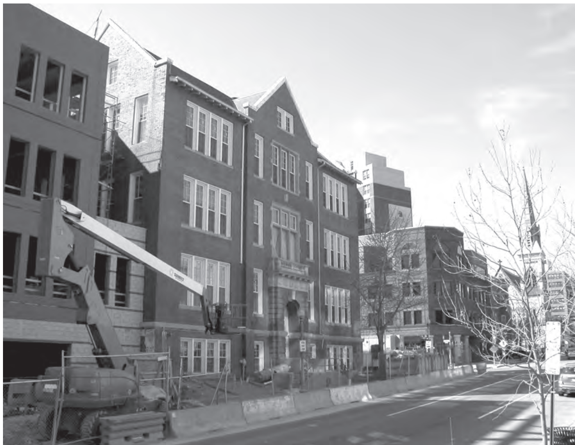
The Corps has made extensive repairs and built additions to the Thomson Elementary School in downtown Washington at 12th and L Streets, NW, which was scheduled to reopen for the 2005–06 school year. Photograph by Darren Santos
