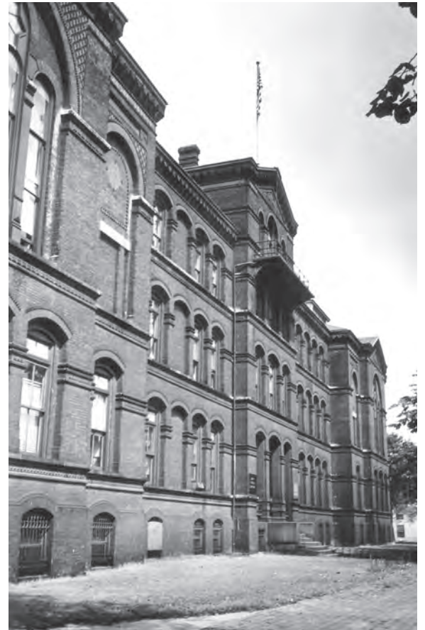
Adolf Cluss's 1885 design for the Army Medical Museum, located on the Mall's south side at 7th Street, SW, was built by Colonel Thomas Lincoln Casey using inexpensive brick, terra cotta, and iron materials. The building, on the site now occupied by the Hirshhorn Museum, was razed in 1969. (Photographed ca. 1940s)
