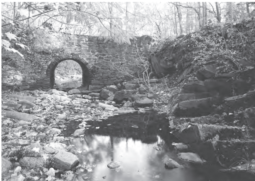
Grant Road Bridge across Broad Branch Creek in Rock Creek Park. Built around 1898, this granite and brick arch bridge twenty-one feet wide and with a ten foot span was one of the earliest bridges that the engineers built in the park. Library of Congress, Prints and Photographs Division, HAER, DC, WASH, 566-2
