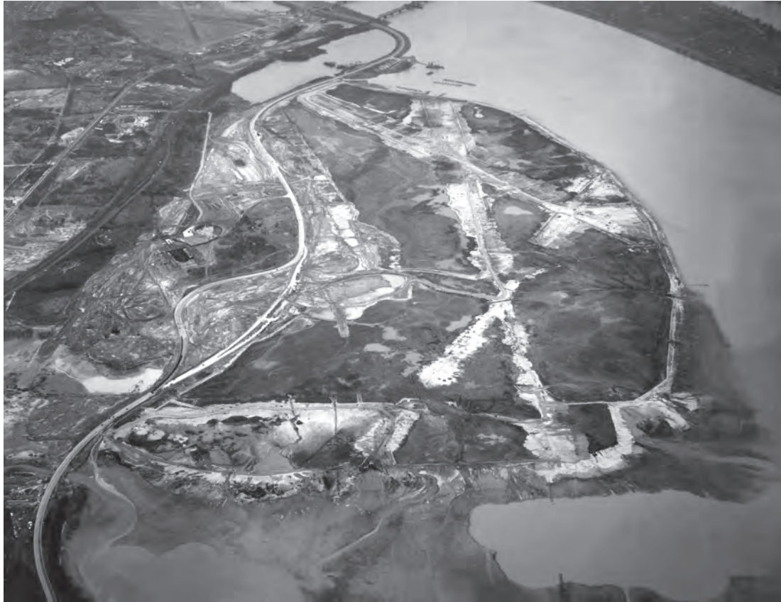
By March 1940 dredging operations were almost completed under the direction of District Engineer Col. Thomas. The Corps paved the four runways seen in this upriver view, landscaped the site, and built hangars and administration buildings. Office of History, Corps of Engineers
