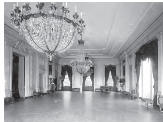
(Top) White House east room under construction, July 1902 Office of History, Corps of Engineers, Restoration of the White House Report
