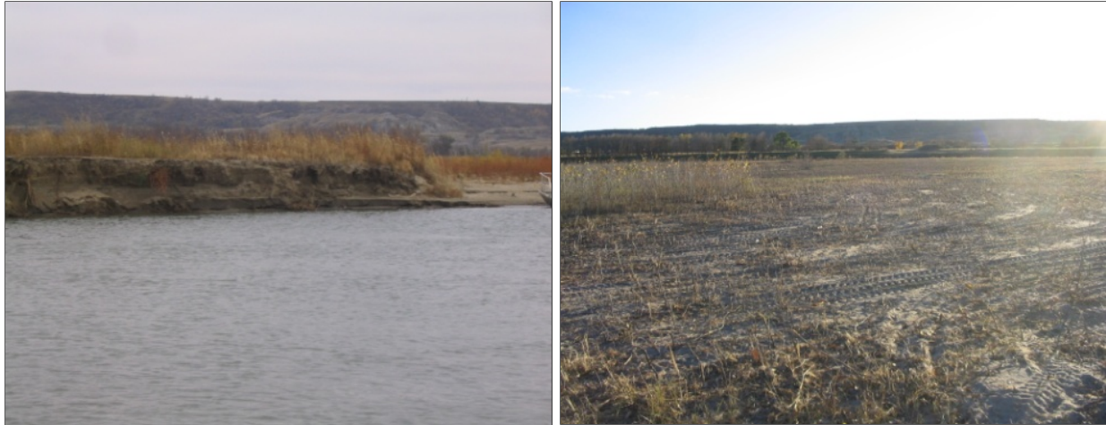
Figure 8. Vegetated sandbar prior to and during removal
