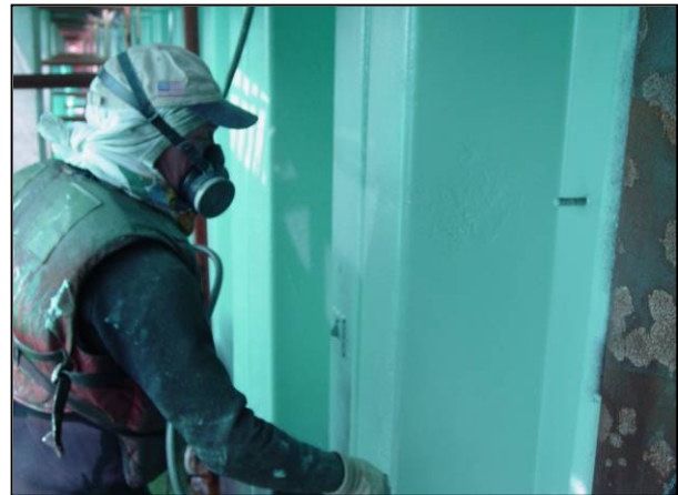
Figure 20. Coating application on San Diego SSP.
