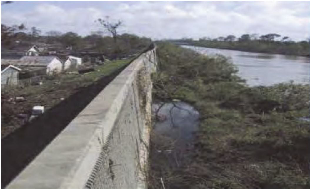
Figure 1. London Avenue Canal floodwall (I-wall) depicting wall deflection failure pattern. The I-wall is composed of concrete wall sections supported by steel sheet piles.
