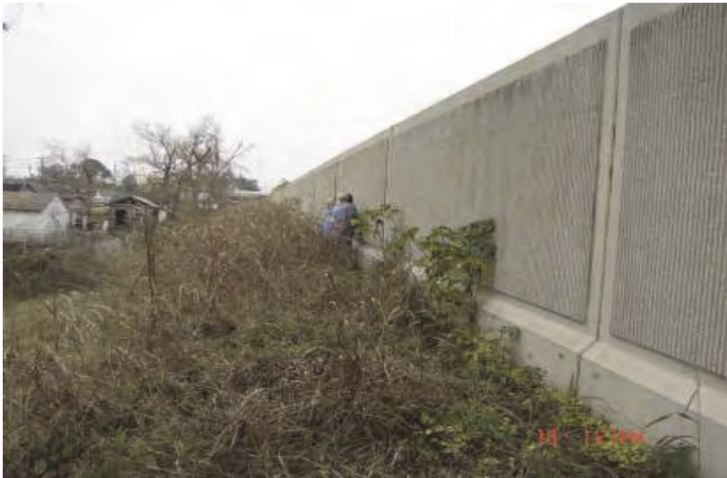
Figure 2. London Avenue Canal I-wall showing joints between panels spaced approximately 30-ft-apart.
