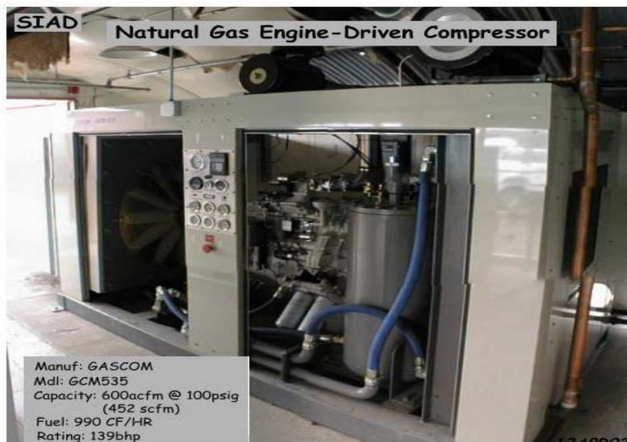
Figure 9. The Ingersoll Rand/MAN NGEDAC, Gascom 635.
