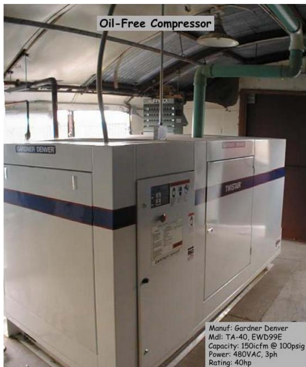
Figure 10. Gardner Denver TA-40 oil-free breathing air compressor.
