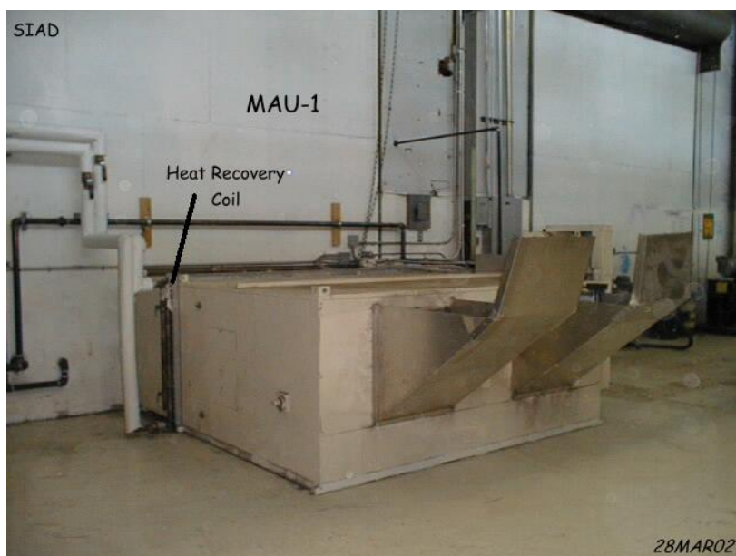
Figure 14. MAU-1 heat recovery coil.
