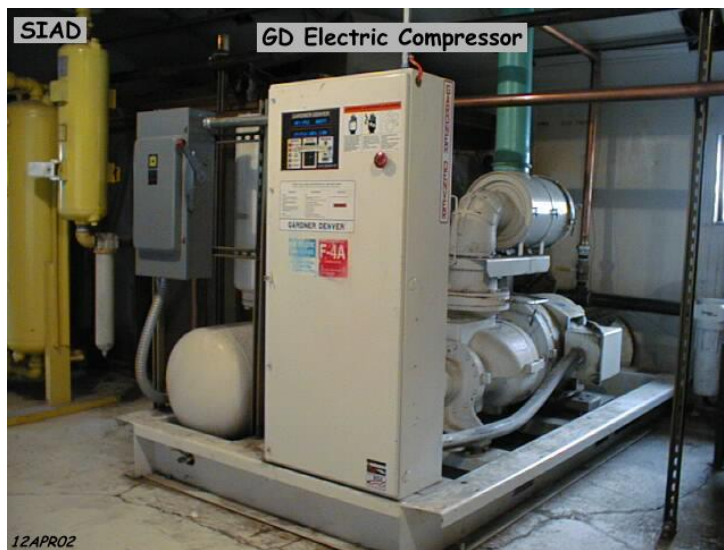
Figure 11. Backup Gardner Denver electric compressor.
