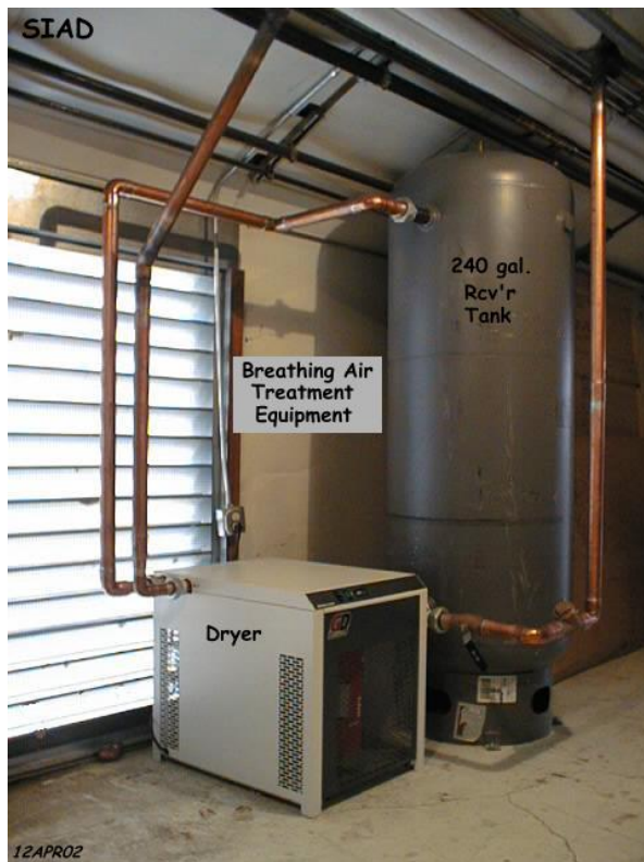
Figure 13. Oil-free compressor receiver and dryer.
