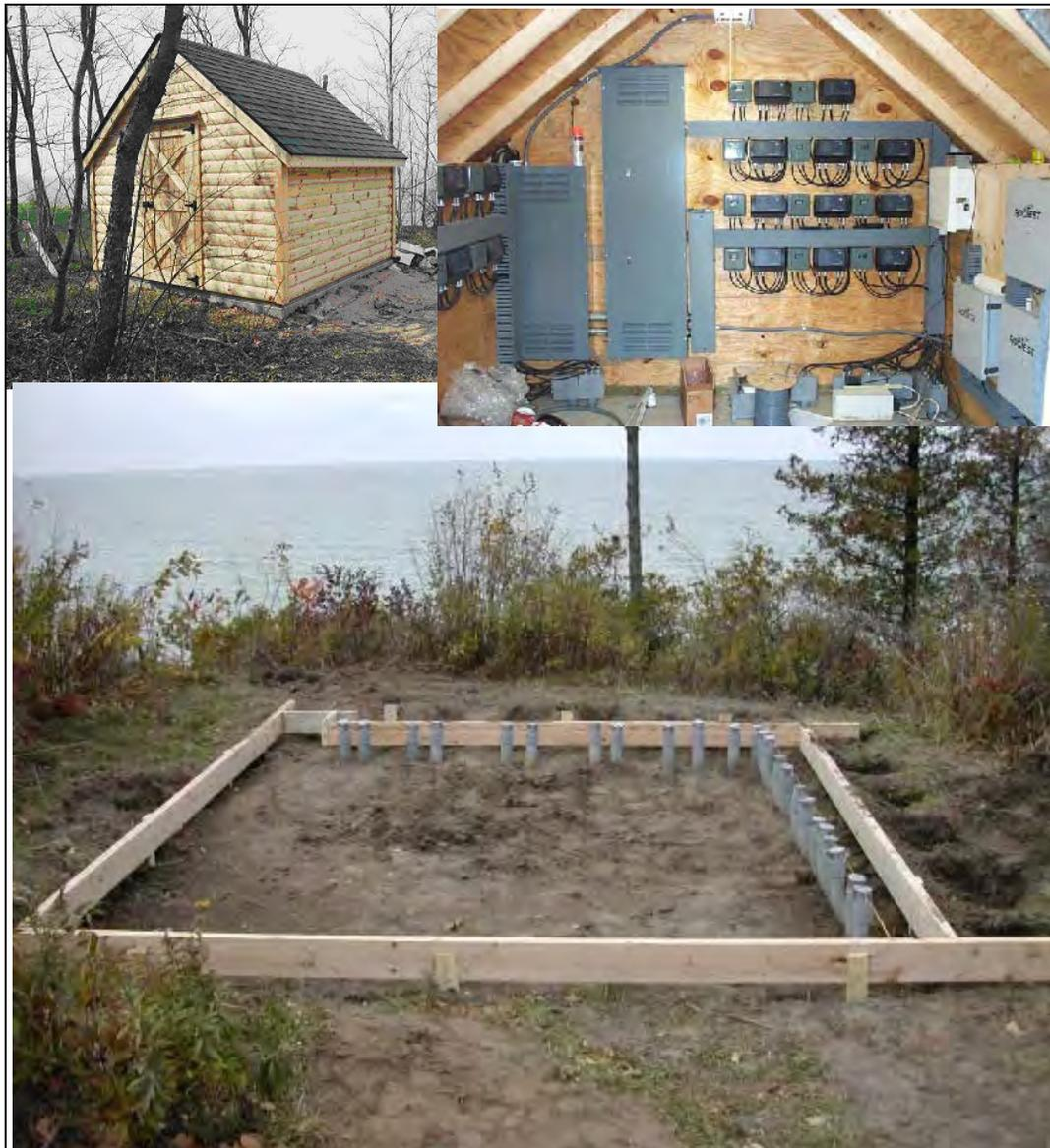
Figure 29. Data-control shed, clockwise from top left, atop each bluff site; pump and instrument control boxes and DAUs inside shed; and construction of shed foundation showing buried conduits for instrumentation wiring.
