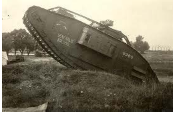
Figure 6. A Mk V Tank Crossing a Trench (From “Mk V Walkaround”)
