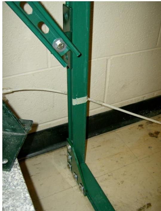
FIGURE 6.1-2: CORNER CONNECTION OF BEACON FRAME WITH DIAGONAL SUPPORT BAR
