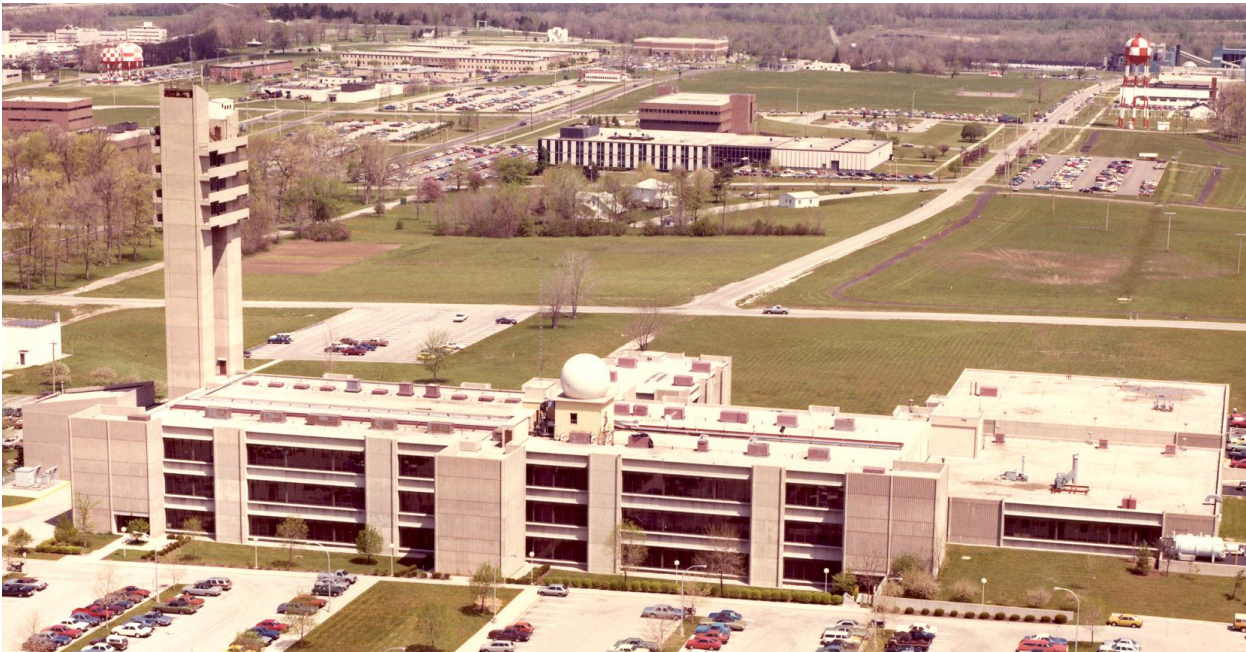
Figure 2 AFAL's Original Rooftop Facility on Building 620
