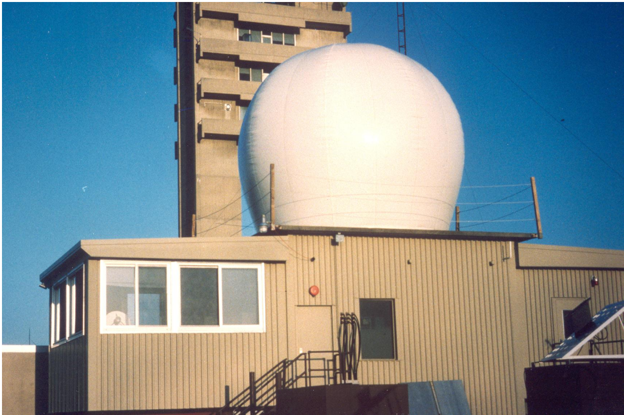
Figure 3 Upgraded Rooftop Facility
