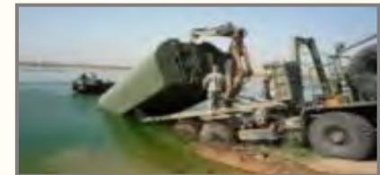
Improved Ribbon Bridge
