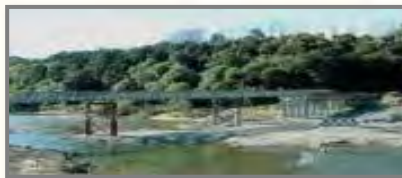
Bailey Bridge (L)
