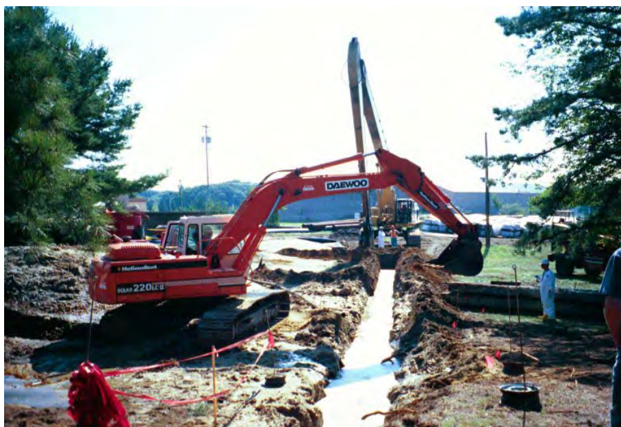
Figure 5-3. Guar slurry used during biopolymer PRB construction.
