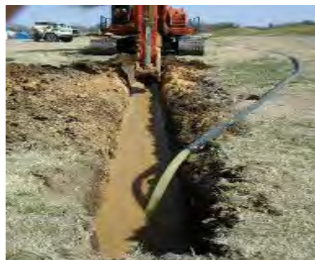
Figure 6-4. Biopolymer trench construction.
