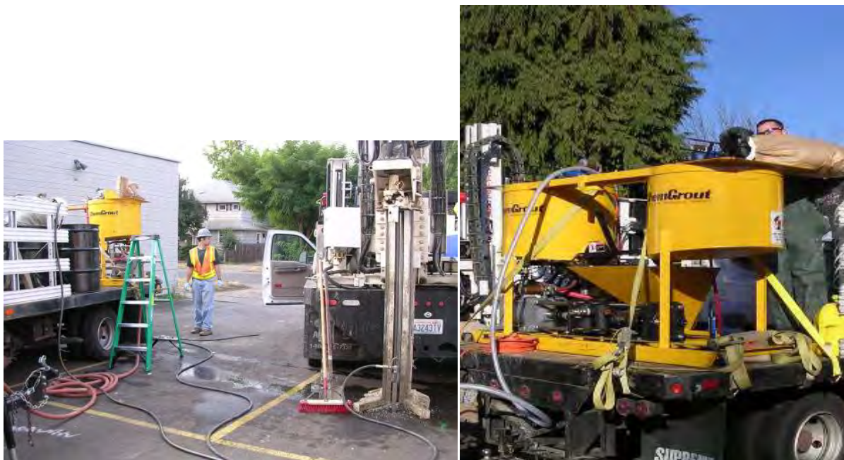
Figure 4-7. EHC mixing and injection equipment.
