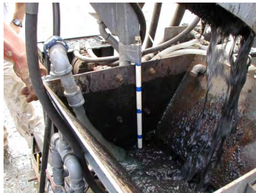
Figure 6-5. Iron guar mixture prepared for direct injection.
