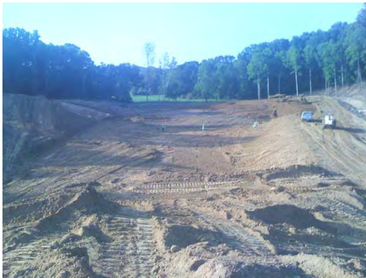
Figure 4.1. Early stage of construction July 2010.
