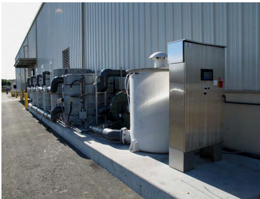
Figure 5-13. Biofilter system.
