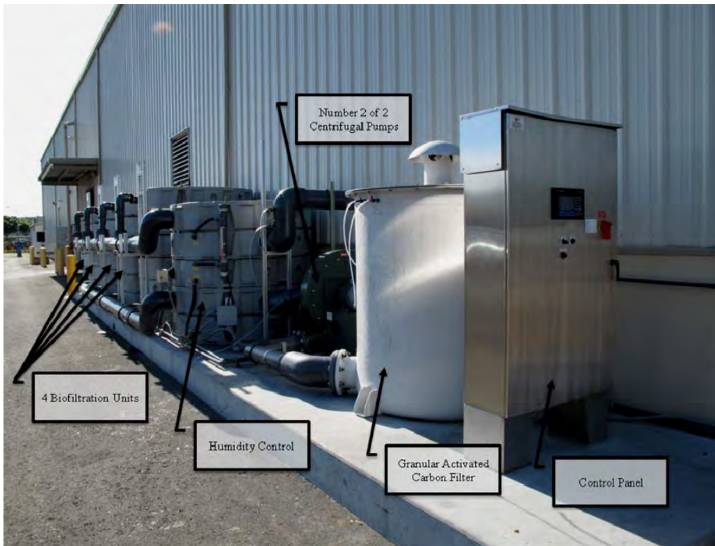
Figure 2-5. Air biofiltration.
