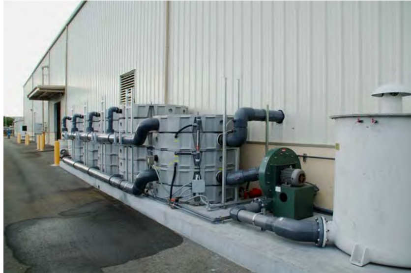
Figure 6-9. Biofilters for treating the exhaust gases of the SBR.
