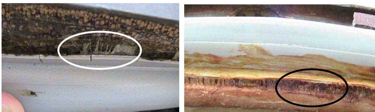
Figure 7. Edge lifting 3M-1357 (left) and 3M-847 (right).
