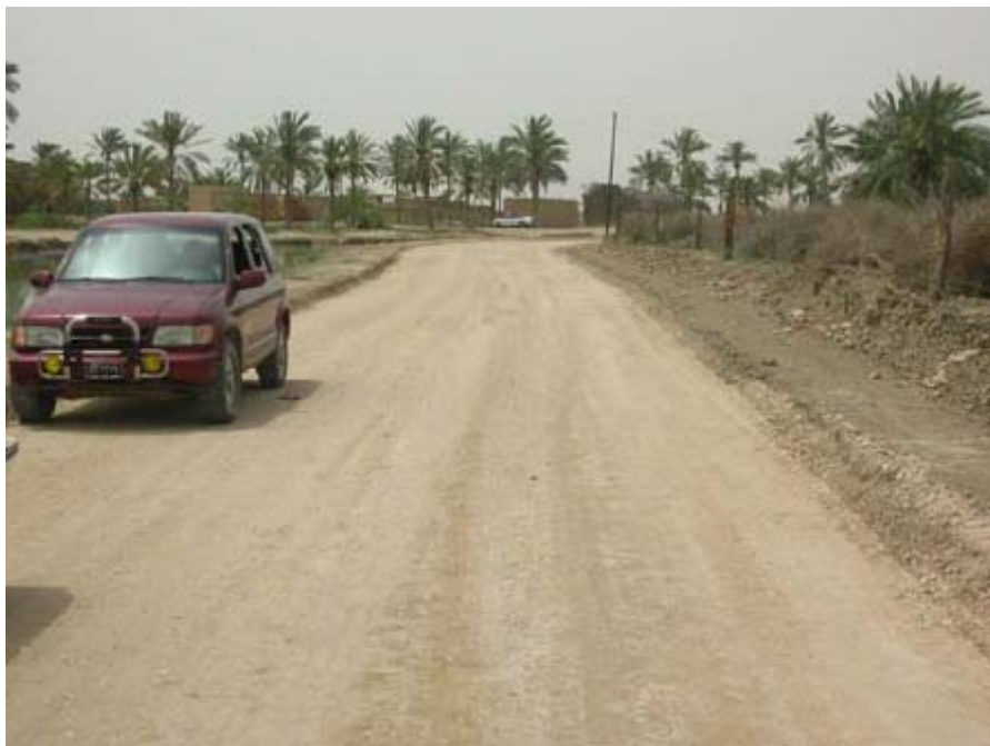
Site Photo 6. Compacted sub-base. (Photo provided by USACE)
