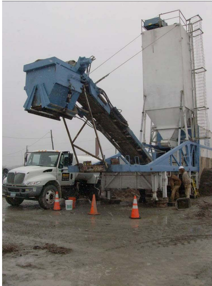
Figure 15. Setting up the ARAN continuous mixing pug mill.
