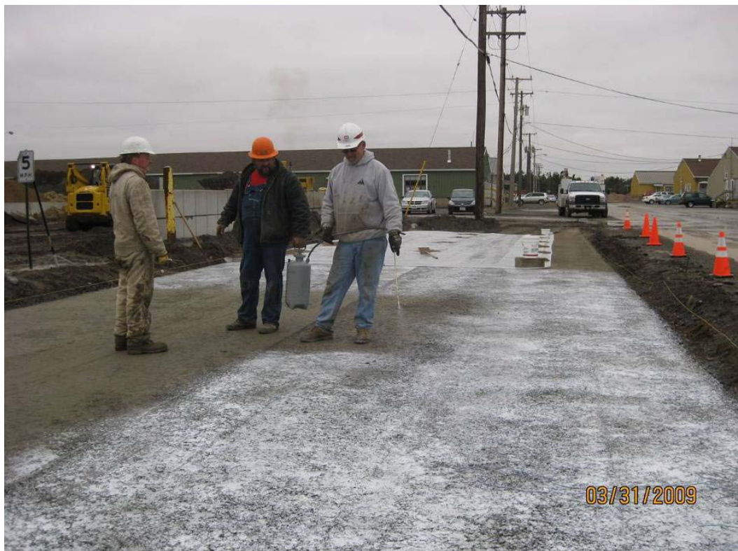
Figure 27. Applying curing compound and plastic sheathing to completed test lanes.
