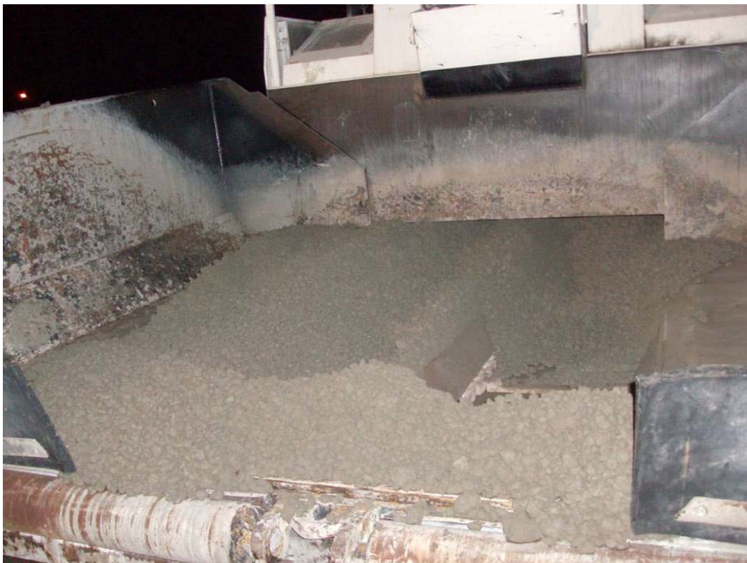
Figure 25. Fresh cold-RCC mixture placed in paver.
