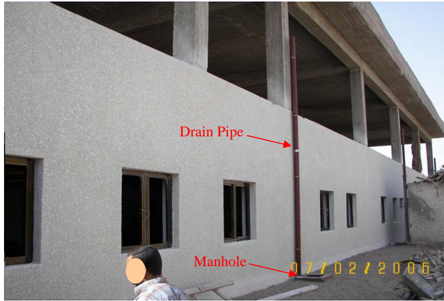
Site Photo 13. CCU exterior with downspout feeding into sewer manhole.
