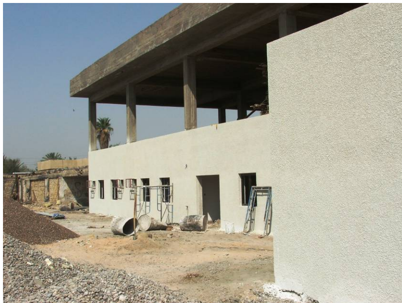
Site Photo 6. Exterior walls of the CCU after plastering and rendering.
