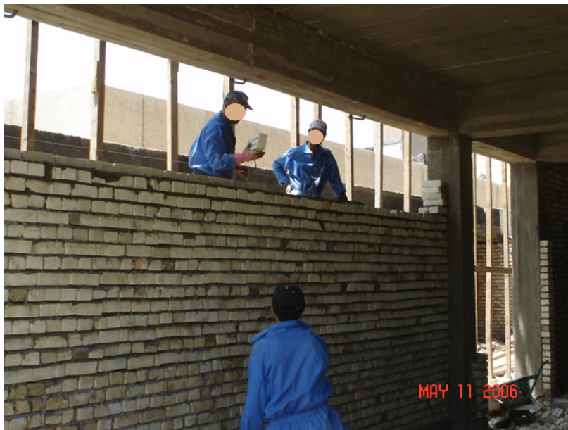
Site Photo 5. Exterior wall brick work (Photo provided by USACE)
