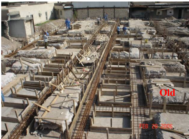
Site Photo 2 - Wall footings and tie beams under construction (Photo provided by USACE)
