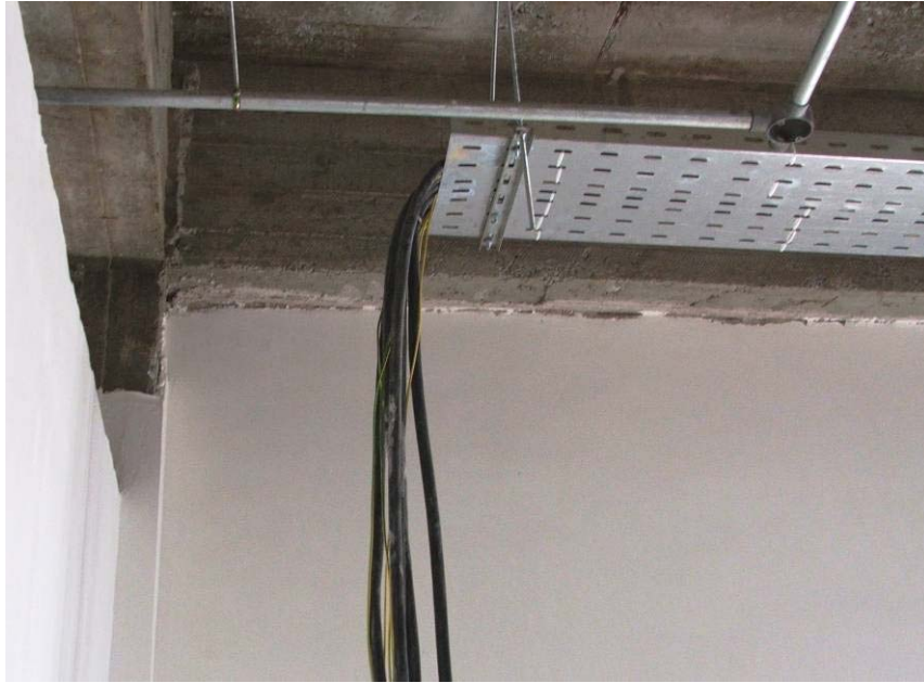
Site Photo 12. Cable tray and cable to connect the main distribution panel.
