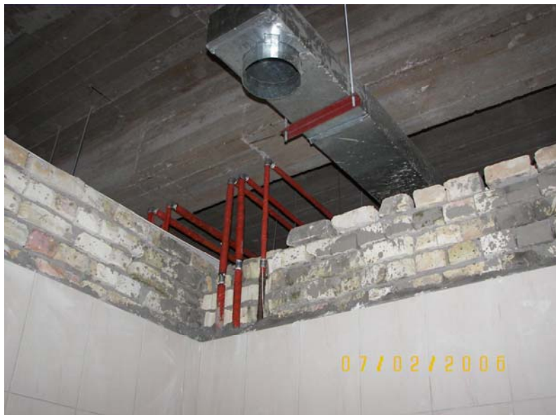
Site Photo 9. Water lines and exhaust system ductwork above one of the patient bathrooms
