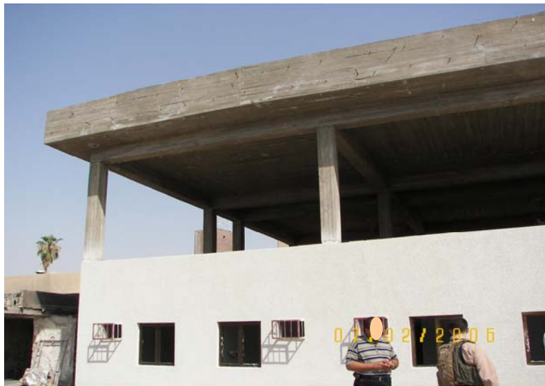
Site Photo 14. First floor columns and beams supporting roof
