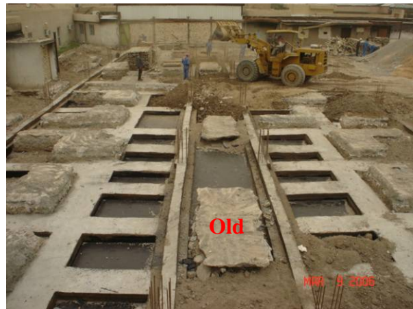
Site Photo 3 - Completed wall footings and tie-beams (Photo provided by USACE)
