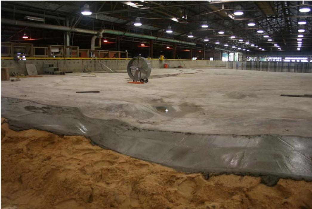
Figure 11. Newly cast section of the Small-Area Model upstream of the Port of Anchorage.
