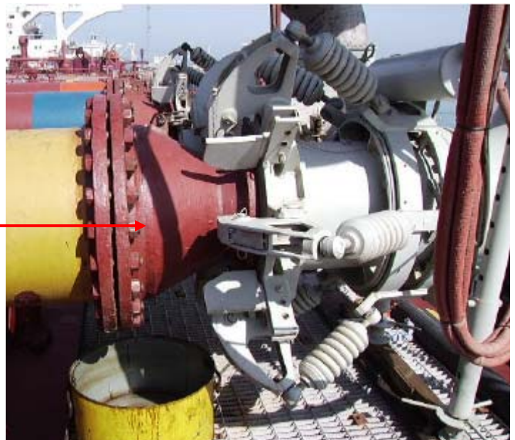
Site Photo 18. Connection of loading arm to receiving tanker
