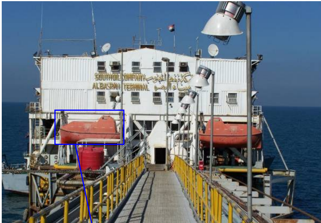
Site Photo 20. Existing two enclosed evacuation escape capsules
