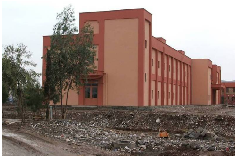
Site Photo 8. Exterior of new barracks facility
