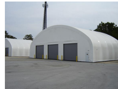
Controlled Humidity Protection
