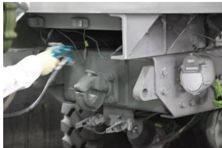
Zinc-rich Paint Application to LVS Trailer
