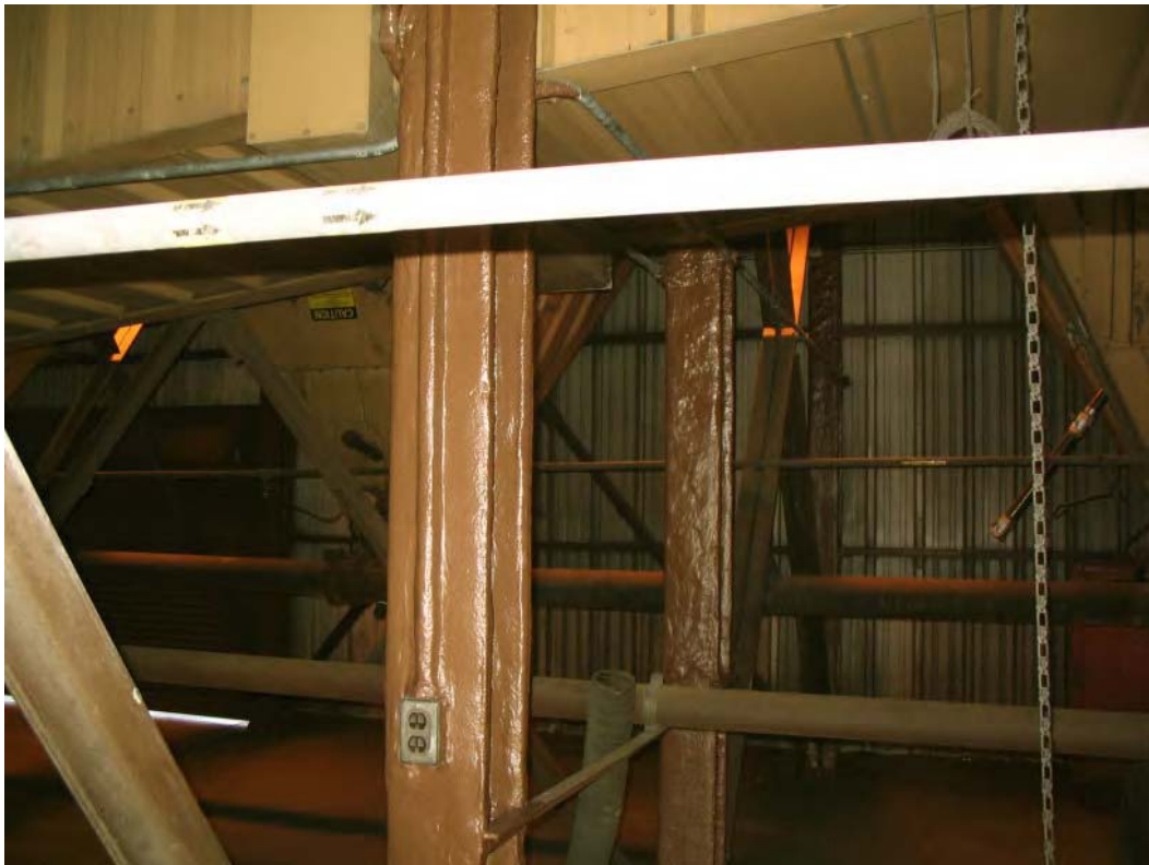
Figure 4. Building 227 interior after coating application.
