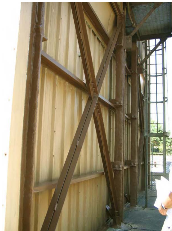
Figure 3. Building 227 exterior after coating application.
