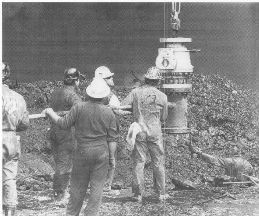
Oil well firefighters cap an oil well.
