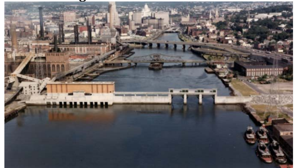
Figure 2. Fox Point Barrier
