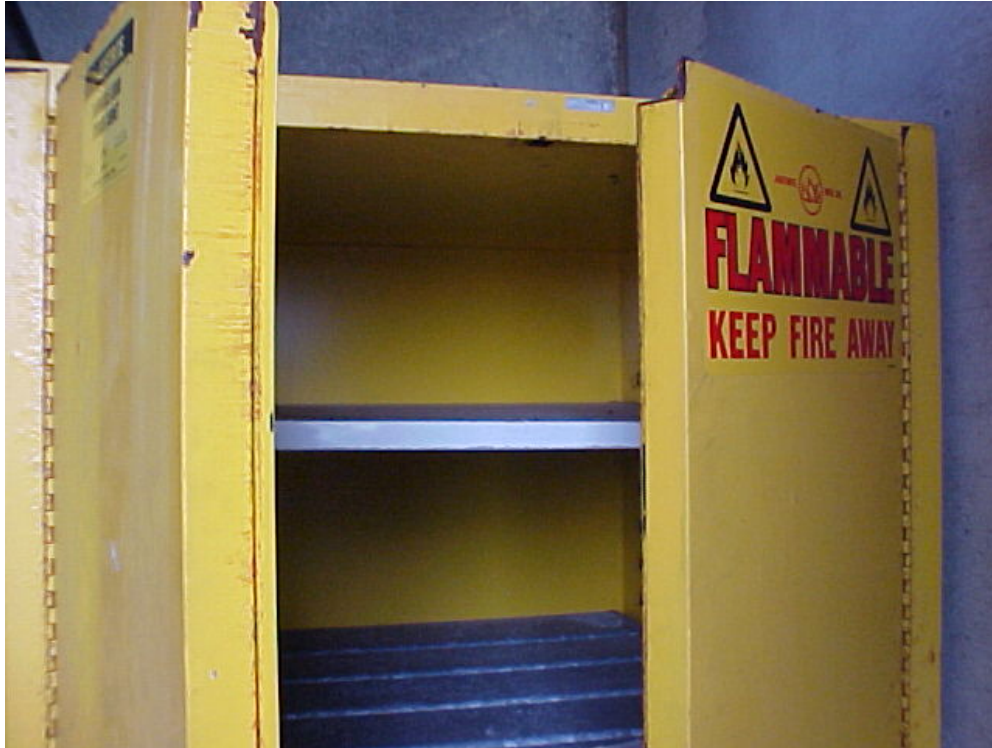
Photograph 57: Empty flammables storage cabinet inside the Hazardous Materials Building #006. View looking east.
