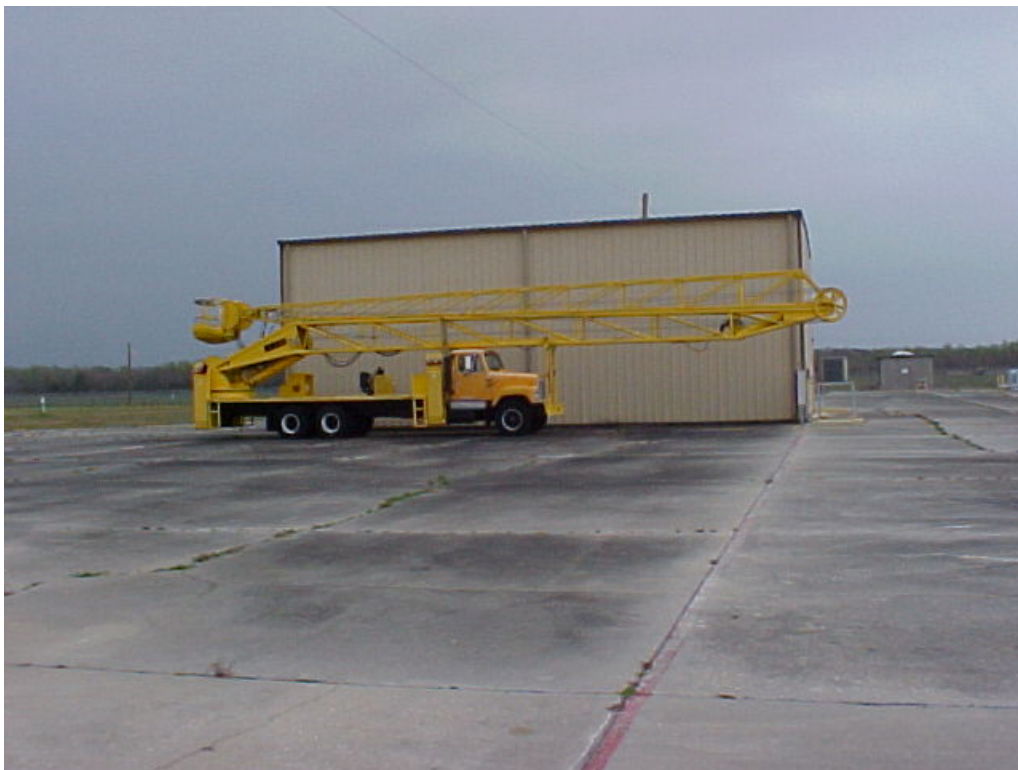
Photograph 47: West-facing wall of the Payload Service Building #003 and the vehicle crane used for balloon maintenance.
