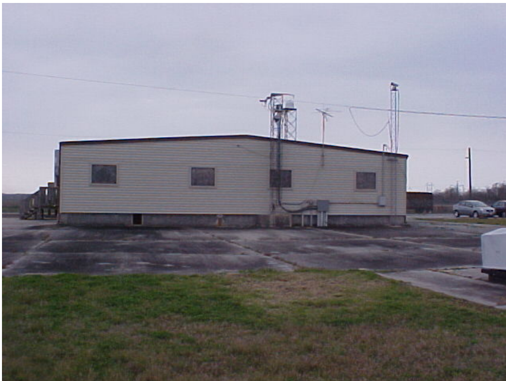
Photograph 5: North wall of the Operations Building #001.
