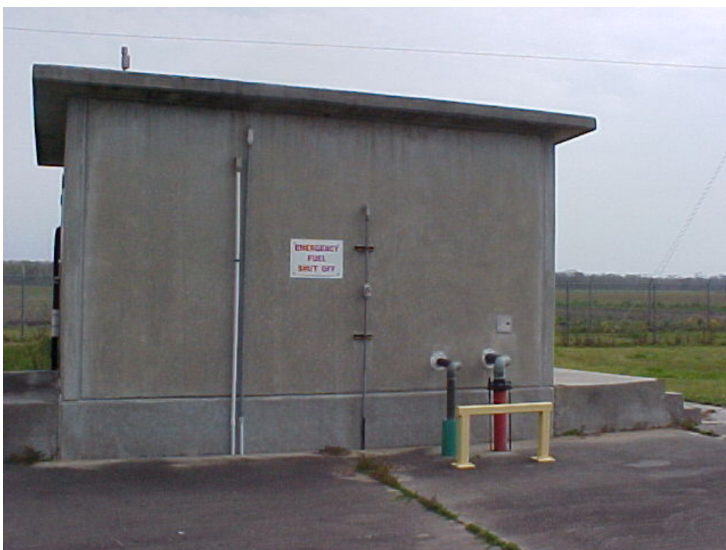
Photograph 62: West-facing wall of Pump House. View is looking east.
