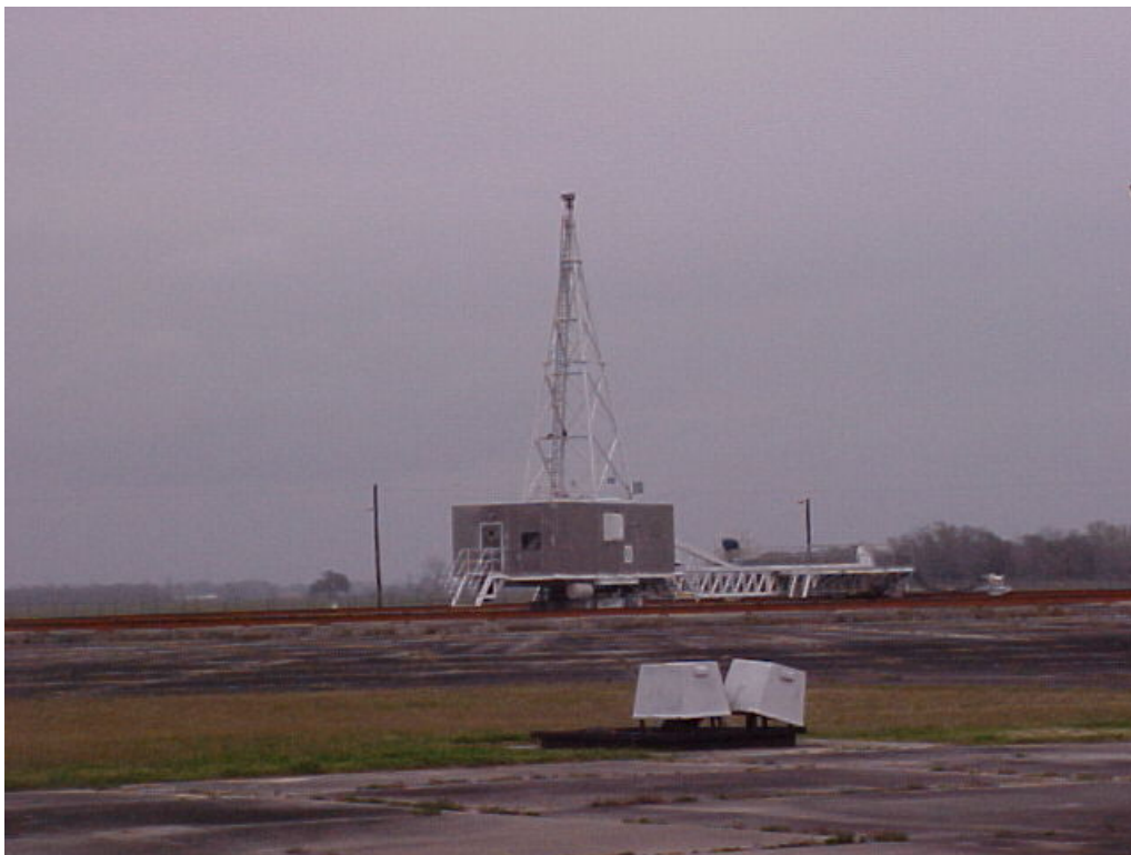
Photograph 71: Tether and mooring rail in background. Wastewater treatment plant in the foreground.
