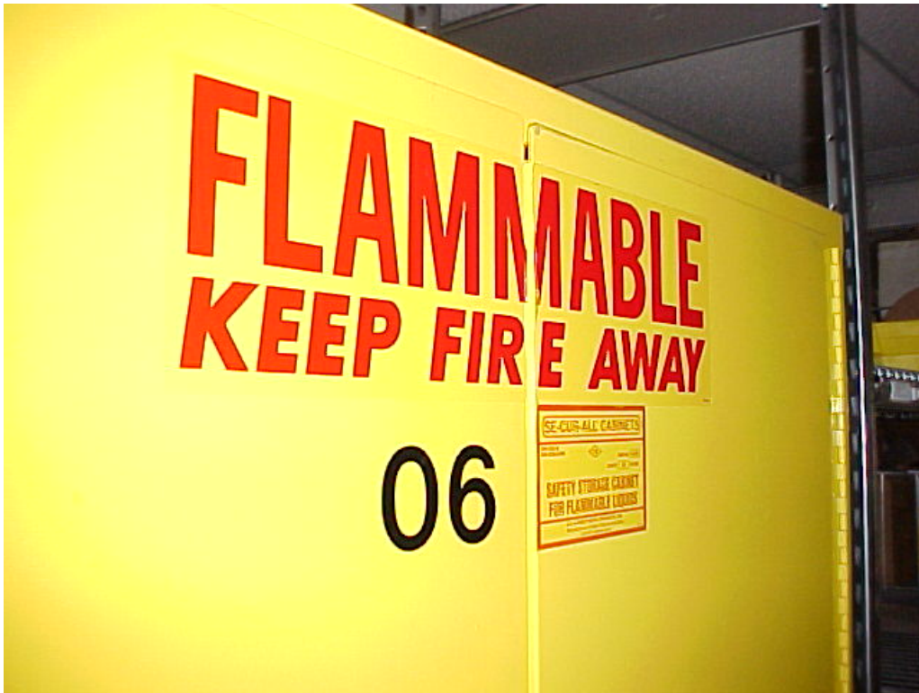
Photograph 9: Flammable storage cabinet in the Operations Building #001.
