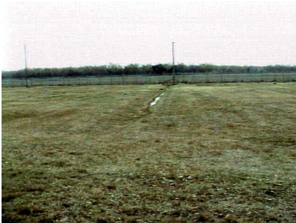
Photograph 70: Drainage swale for the wastewater treatment plant. View is looking east from the launch pad. Sugar cane fields are located beyond fence line.
