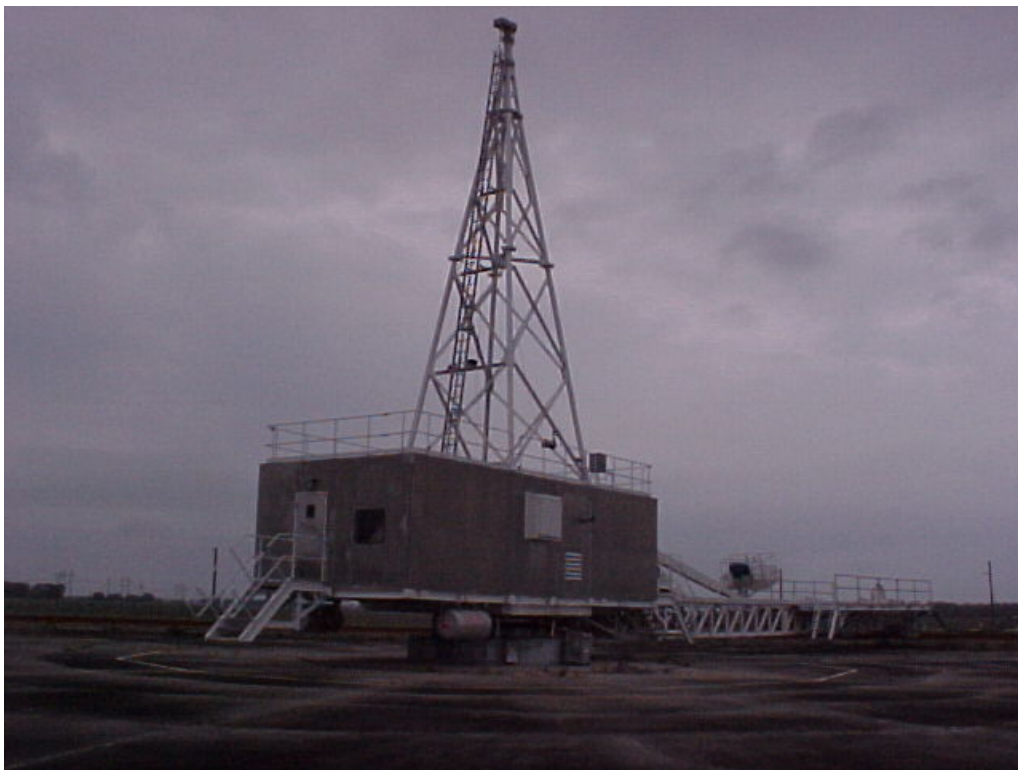
Photograph 73: Additional photo of the Tether Building.
