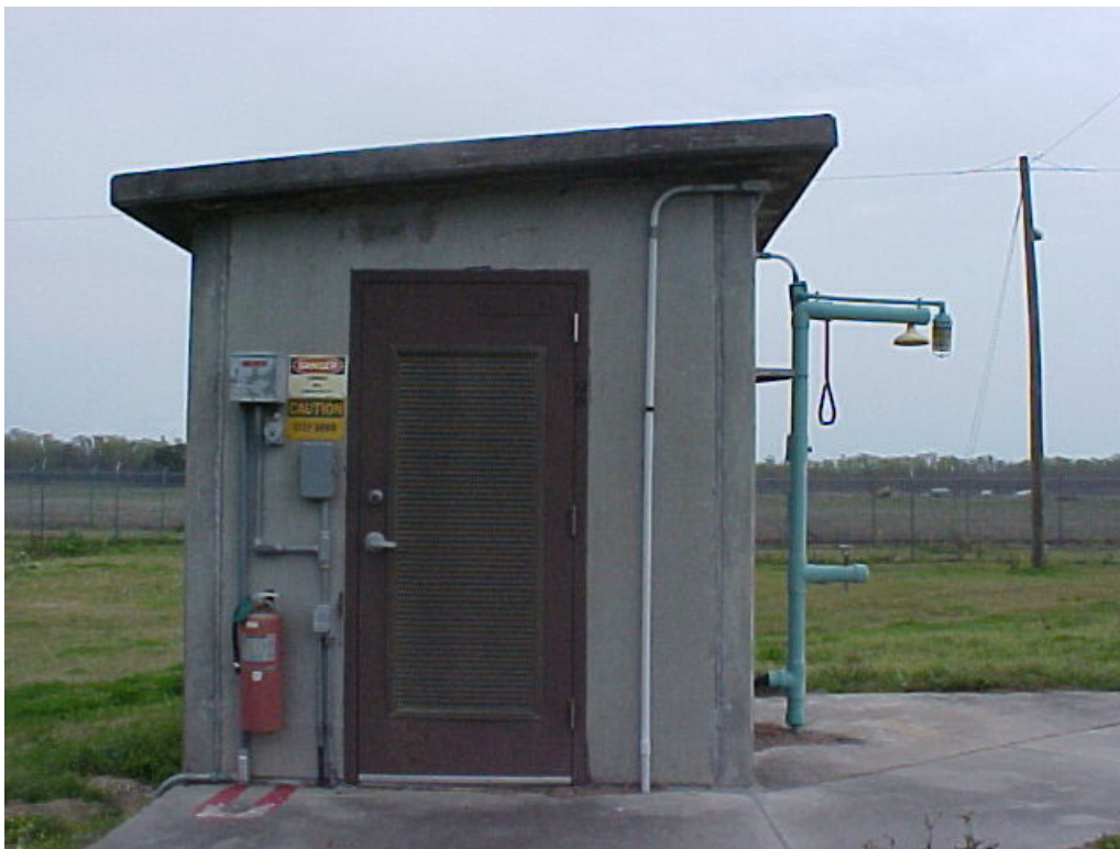
Photograph 55: Hazardous Materials Building #006 exterior. View is looking east.
