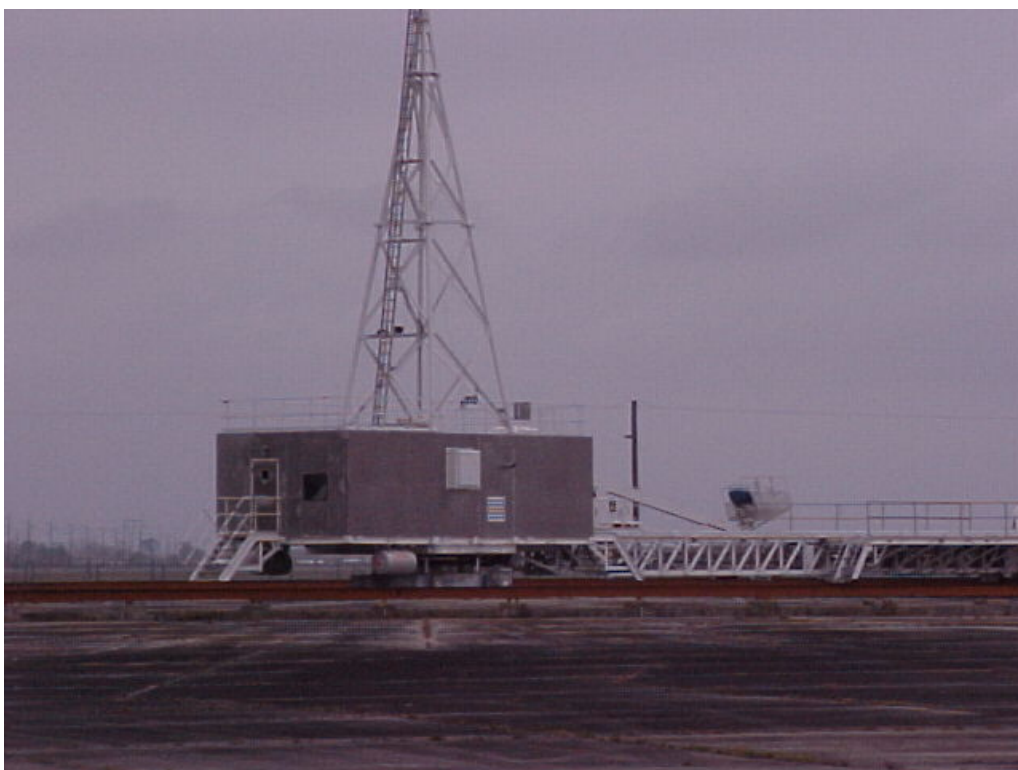
Photograph 72: Closer view of Tether Building and mooring rail.
