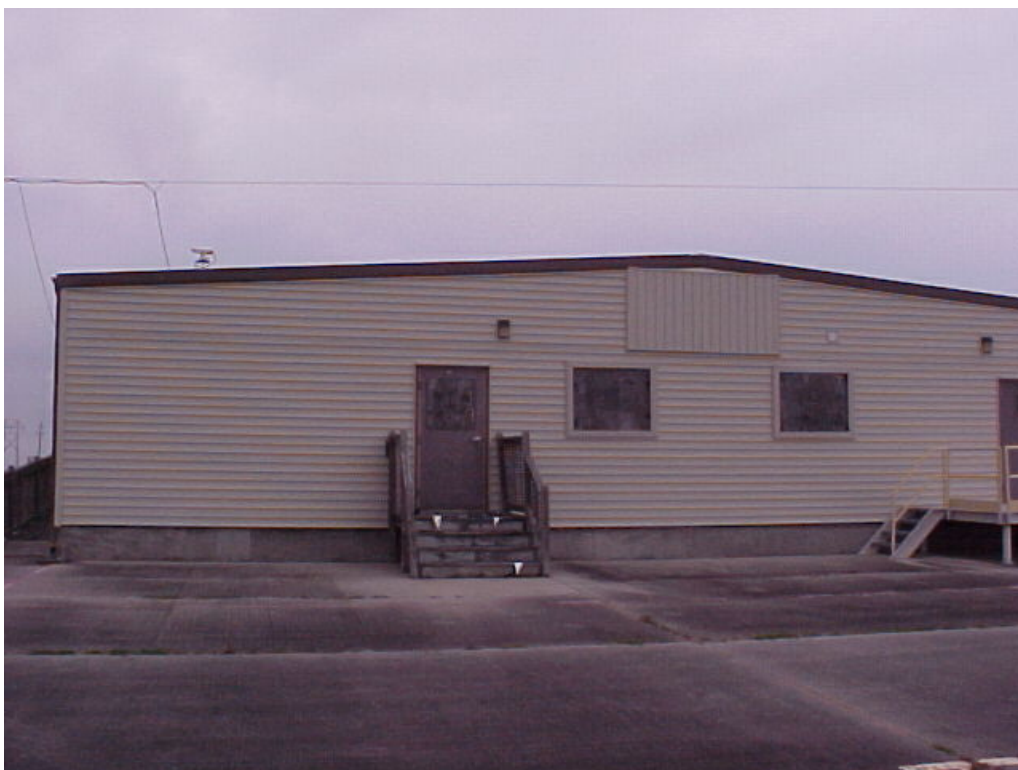
Photograph 3: South entrance to the Operations Building #001.
