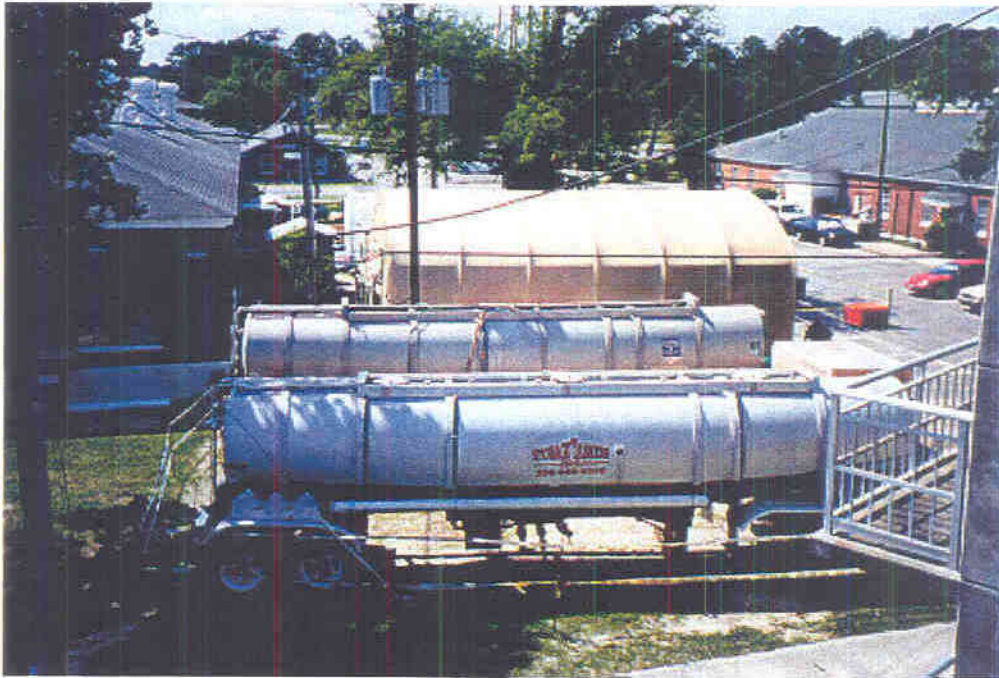
Wastewater tankers for disposal and for contingency
