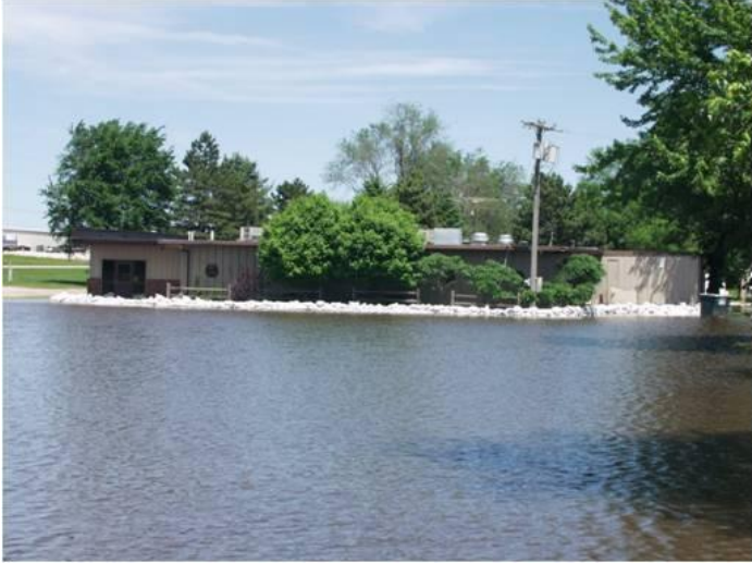
Sandbags held at Cattleman's Restaurant at Belmond, Iowa, 9 June 2008.
