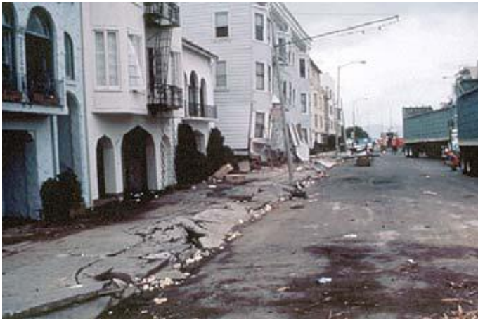
Liquefaction-related damage in the Marina District of San Francisco followed the Loma Prieta earthquake.
