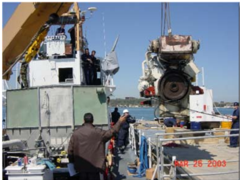
Cutter Engines Changeout
