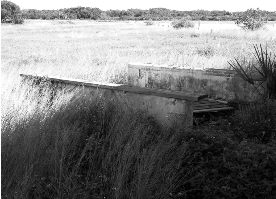
Figure 66. Launch support building cooling tower walls (ERDC-CERL 2007).
