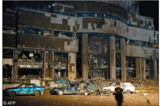
Firemen comb the rubble of the HSBC Bank building in Istanbul after the terrorist attack, 20 November 2003.
