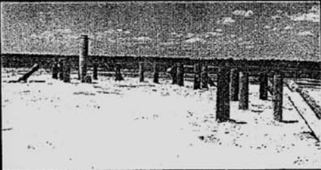
CONCRETE JERSEY BARRIERS AND ENGINEER STAKE JACKS
