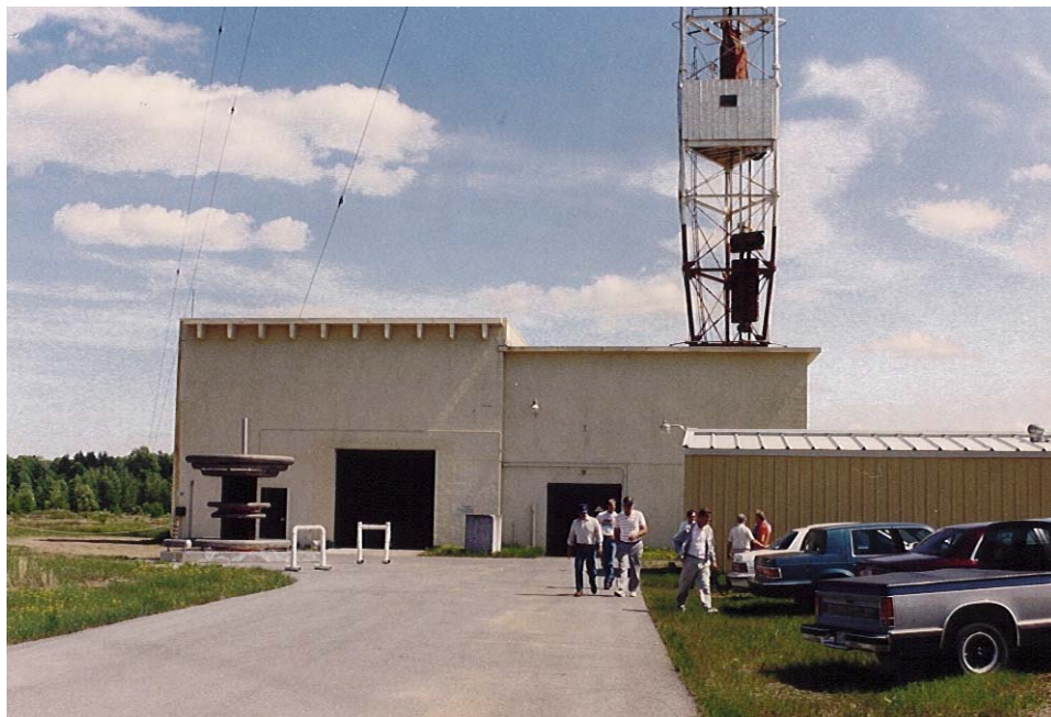
Figure 5-4. High-voltage test area.
