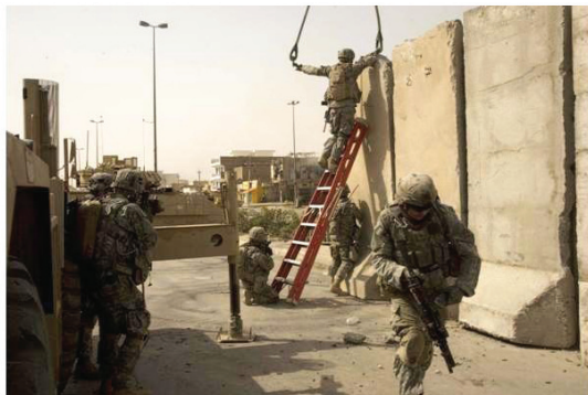
Photo 6: Even with protection from a SEAL sniper team, M1 Abrams tanks, Air Weapons teams, and other infantrymen, the four to six man construction team from Bravo 1-68 IN (attached to Charlie Company 1-68 Armor) came under daily enemy fire from buildings north of PL Gold. From left to right: (just helmet) CPT Boyes, XO/C/1-68; (standing next to helmet) 1LT Poole, XO/C/1-6; (kneeling) PFC Nguyen B/1-68; (on ladder) SPC Ervin, C/1-68; (under ladder) SSG Lewis, C/1-68; (running towards camera) SGT Ziska, C/1-68.
