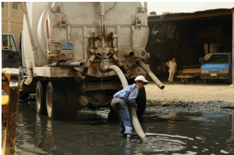
Photo 12: Sewage from pipes damaged by special groups and criminal attacks on the Jamilla Market of the Sadr City district of Baghdad is hauled away by workers to pave the way for infrastructure improvements June 2. As soon as the sewage was removed, underground pipes were repaired and Iraqi workers began working on the road to speed the flow of traffic into one of Baghdad's largest market places. (U.S. Air Force photo/Tech Sgt. Cohen Young)
