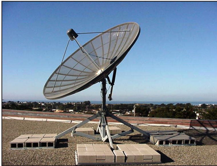
Antenna receiving geostationary satellite data
