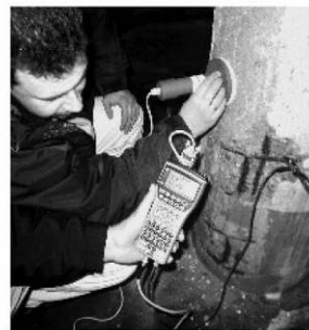
GalvaPulse testing in progress for corrosion activity of a heavily corroded column
