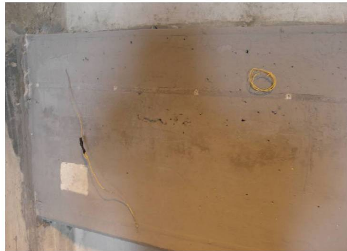
Figure 23. Close up showing titanium mesh connections in sacrificial coating.
