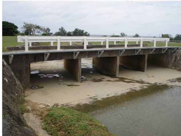
Figure 1. Overview of Culvert #2, looking downstream toward the East China Sea.
