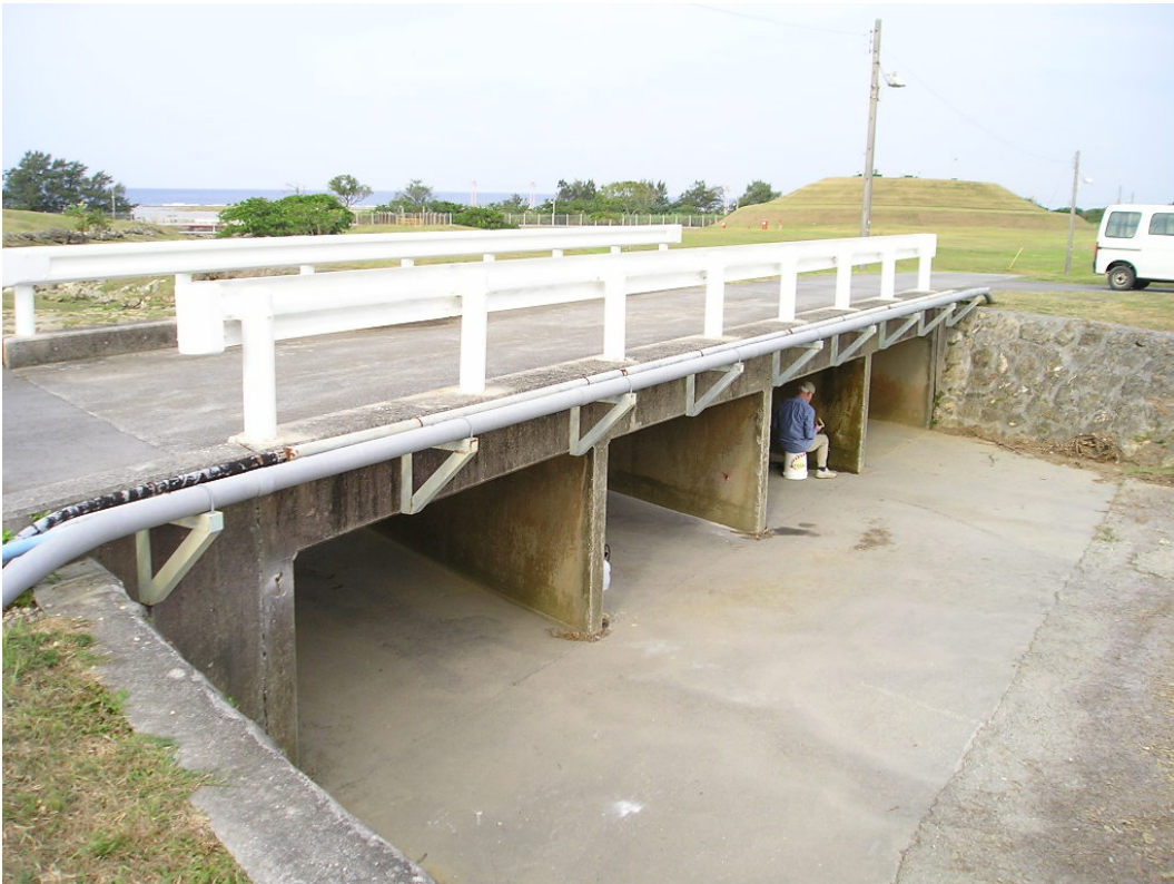
Figure 2.3. Tank farm culvert 2, all concrete surfaces.
