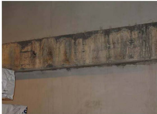
Figure 1c. Closer view of beams "A" before treatment
