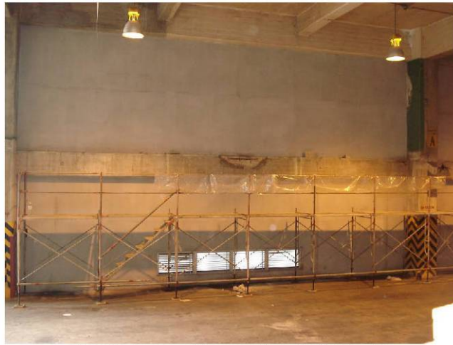
Figure 15. Overview of “Beam 1” at Naha Port Building 306.
