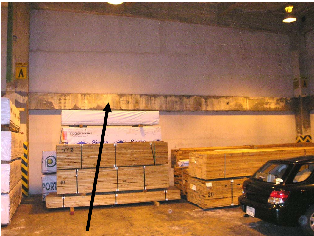
Figure 2.2. Building 306 warehouse, northeast wall, inside ring girder side 2.
