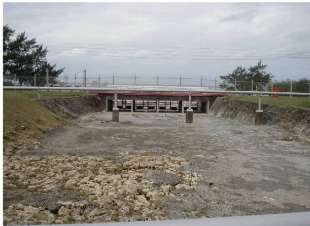
Figure 11. Overview of Culvert #3, looking downstream toward the East China Sea.
