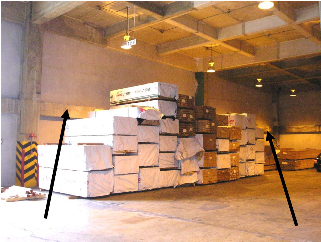
Figure 2.1. Building 306 warehouse, inside ring girder, side 1 (left) and side 2 (right).
