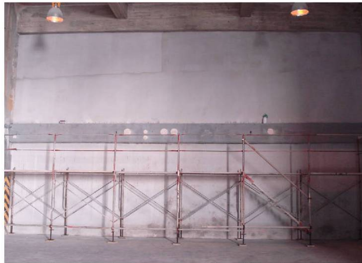
Figure 22. Overview of Beam 2 with the NASA sacrificial coating applied.
