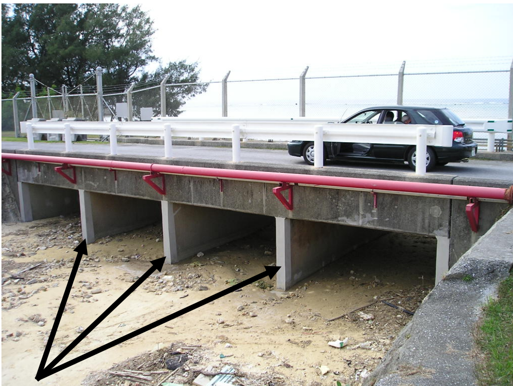
Figure 2.4. Tank farm culvert 3, vertical concrete support components.
