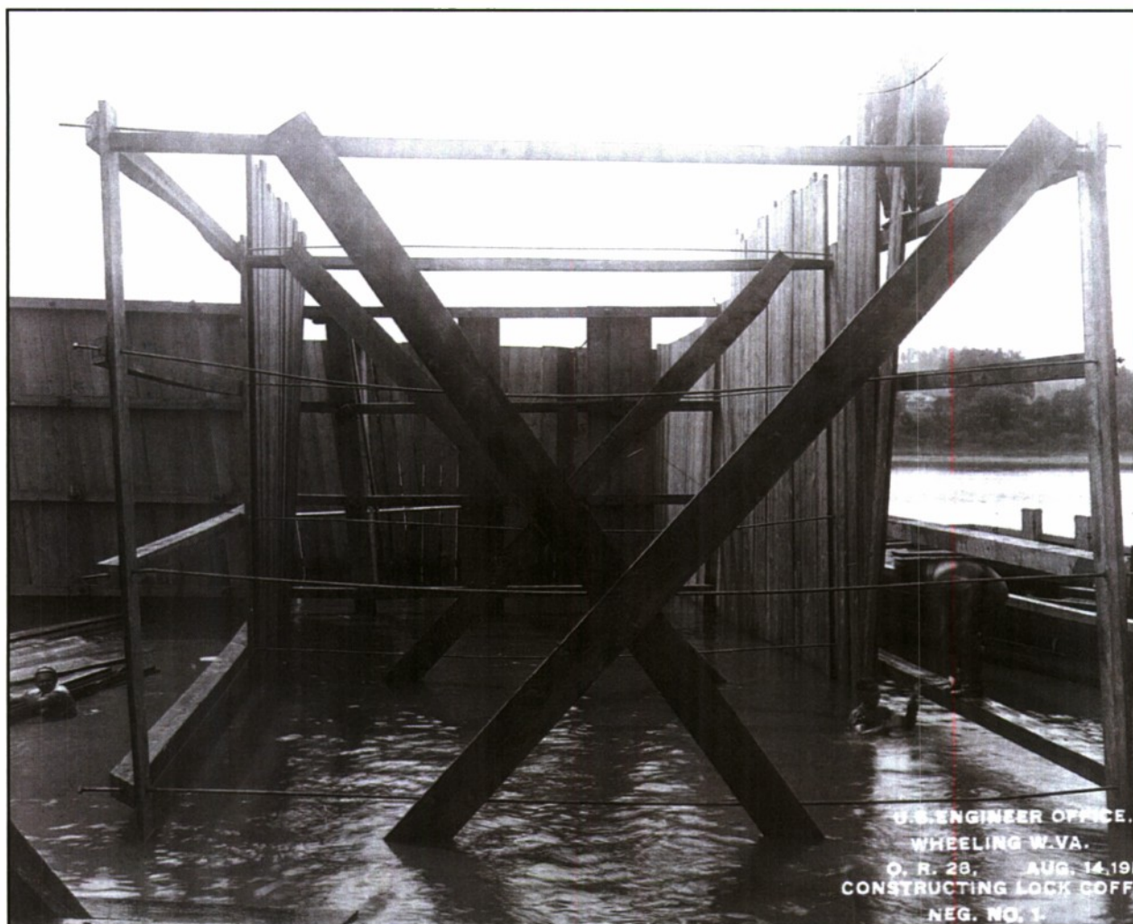
Plate 3. Constructing lock cofferdam. Placing the sheet piling for an Ohio River type box cofferdam. Note the lightness of the construction and the men in the water. August 14, 1911. RG 77-RH, Box 127, Ohio River L/D #28 – Lock/Lock Cofferdam Folder, NARA.
