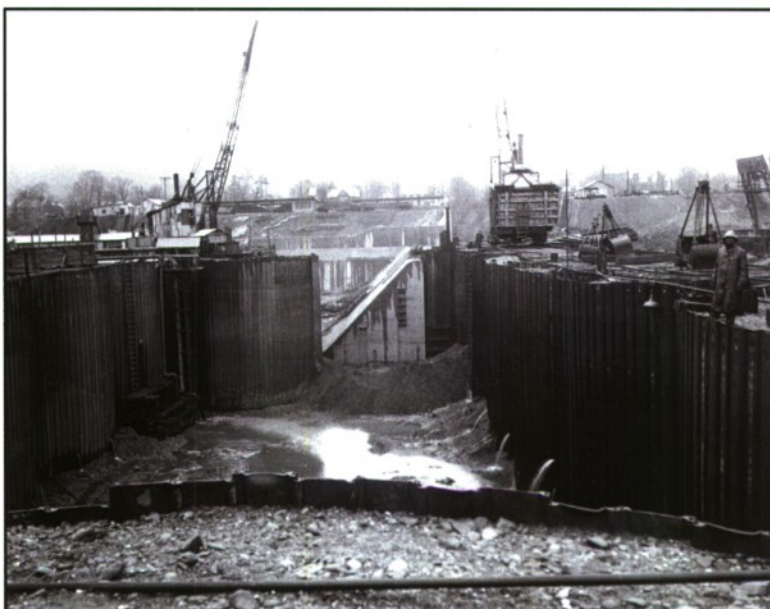
Plate 13. Dashiels Locks and Dam, Ohio River. View toward right shore of cofferdam. 1 October 1928. Photo 5375, Folder 3, Ohio River Dashiels L/D Photographs 1927, Pittsburgh District, USACOE.
