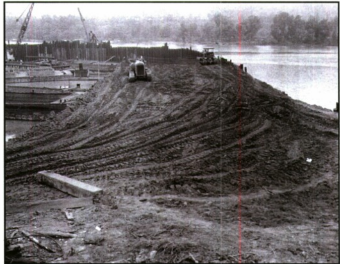
Plate 17. Montgomery Locks and Dam, Ohio River. Placing fill in upstream arm of cofferdam. Note the use of bulldozers to distribute the fill. 15 July 1932. Photo 6570, Ohio River – Montgomery L/D Photographs – 1932 – June 1934, Pittsburgh District, USACOE.
