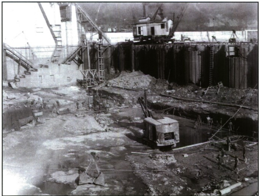
Plate 27. London Locks and Dam, Kanawha River. View of second dam cofferdam. Note the steel pile cofferdam cells and the whirley crane mounted atop the cofferdam. 2 November 1933. RG 77-RH, Box 47, London L/D. Dam and Cofferdam Folder, NARA.
