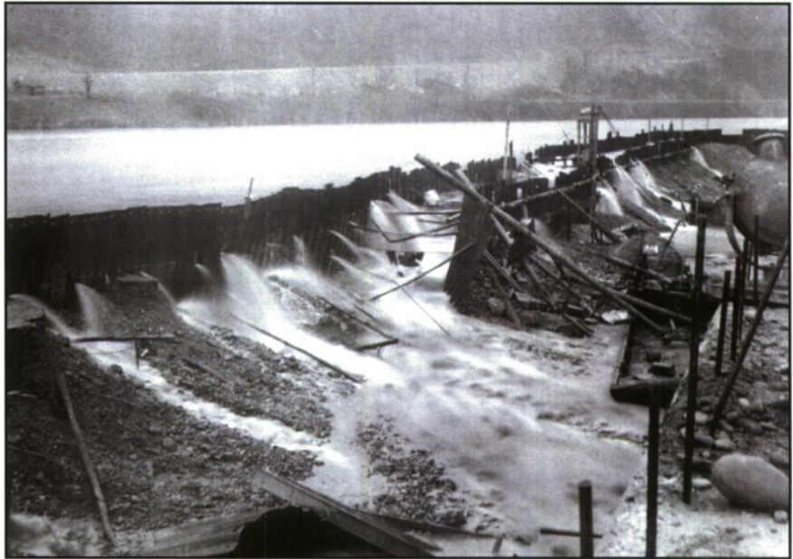
Plate 26. London Locks and Dam, Kanawha River. Collapse of river arm of Lock A cofferdam. The inner wall of sheet piling has failed and the cofferdam fill is sloughing out into the work area as the outer wall of piling fails. 4 February 1932. RG 77-RH, Box 47, London L/D, Lock and Lock Cofferdam Folder, NARA.
