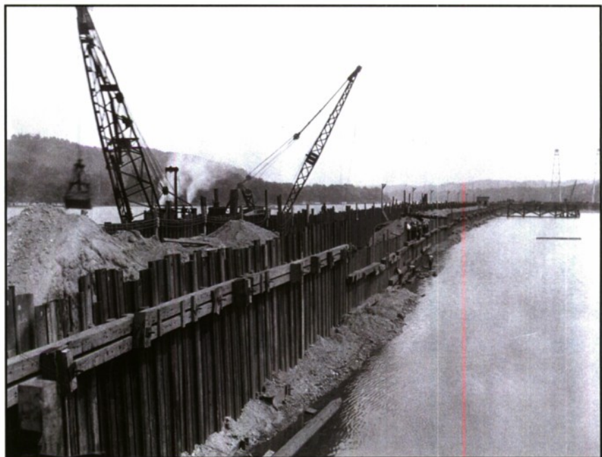
Plate 18. Montgomery Locks and Dam, Ohio River. River arm of steel sheet pile box type cofferdam under construction. Cranes are placing fill within the cofferdam. Note the timber wales and tie rod connections on the outside face of the sheet piling. 17 August 1932. Photo 6619, Ohio River – Montgomery L/D Photographs. 1932 – June 1934. Pittsburgh District, USACOE.
